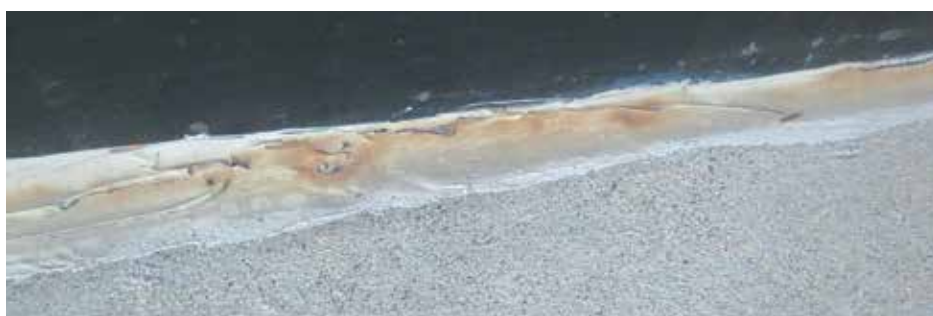
Figure 2. Example of discolored in-service silicone sealant in contact with bitumen-based waterproofing.
