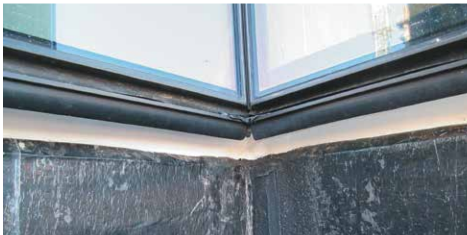
Figure 1. Example of in-service silicone sealant installed in joint between bitumen-based waterproofing and curtainwall frame.
