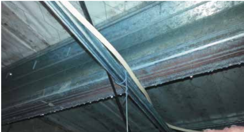
Figure 4. Condensate forming on purlins.
