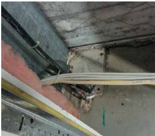
Figure 5. Visible organic growth on the building wrap.
