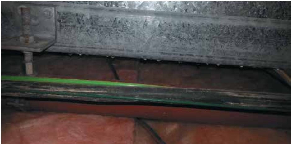
Figure 6. Droplet formation on the steel purlin and rust evident on services bolt and nut.
