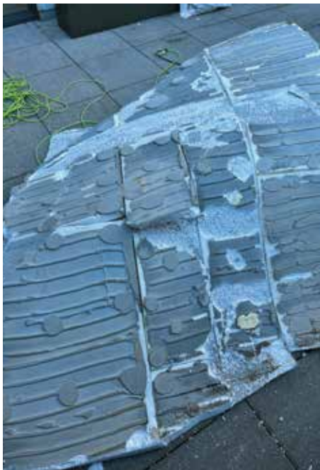
Figure 3. Dollops of adhesive at failure of exterior insulation and finish system.
