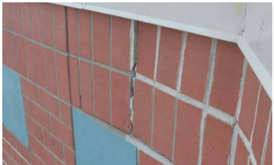
Figure 7. Displacement of brick masonry veneer.
