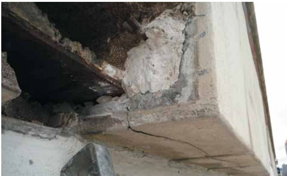
Figure 8. Cracked terra-cotta at corroded beam.
