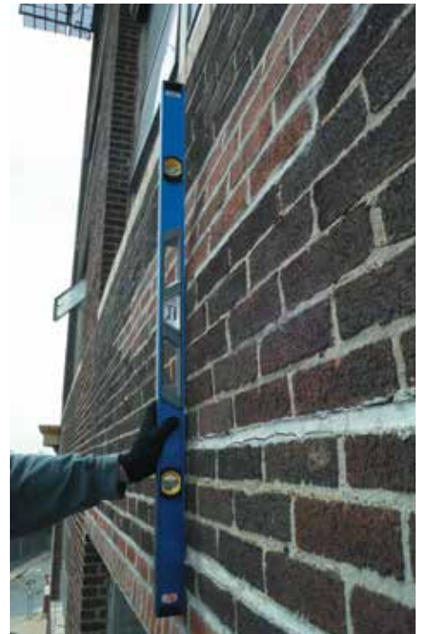
Figure 6. Displacement of brick masonry.
