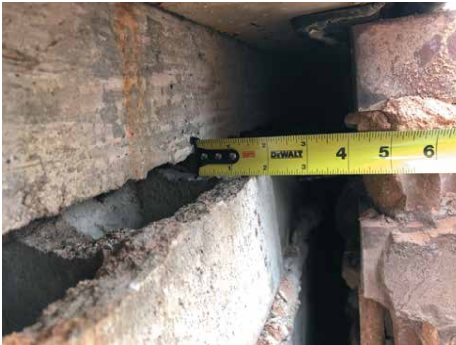
Figure 5. Displacement of backup wall.
