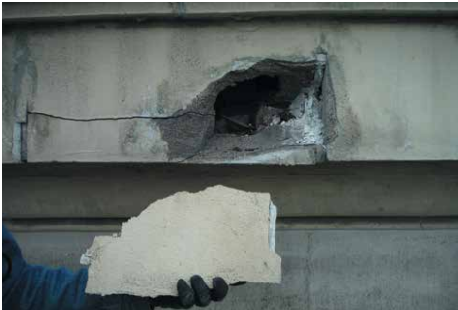
Figure 9. Removed cracked and loose terra-cotta.
