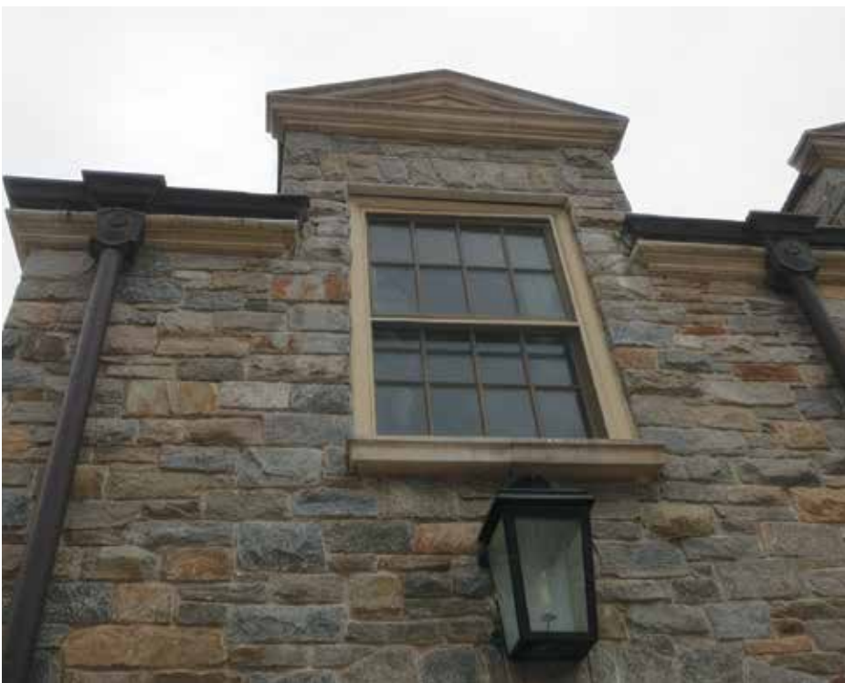
Figure 4. Hung gutter and down leader drainage system.
