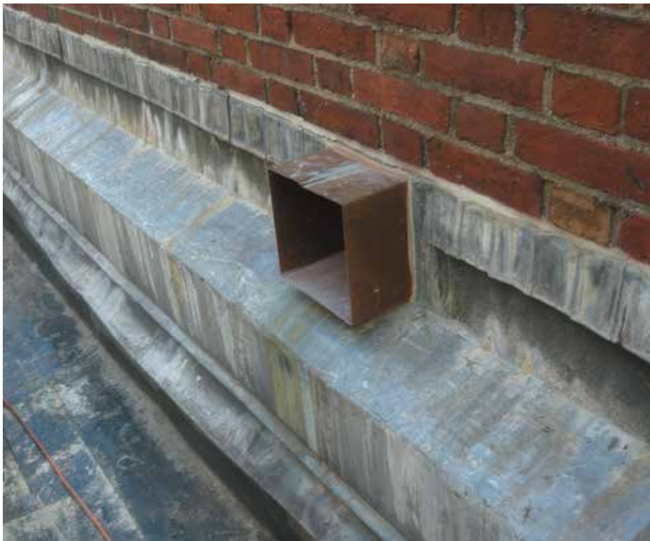
Figure 5. Through-wall scupper drainage system.
