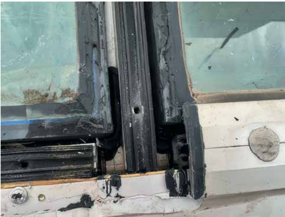
Figure 2. Simple framed skylight with curtain wall framing.
