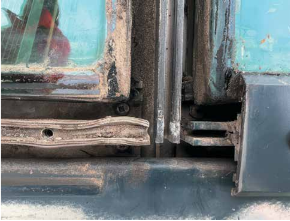
Figure 3. Skylight with overlapped raised drainage channels.
