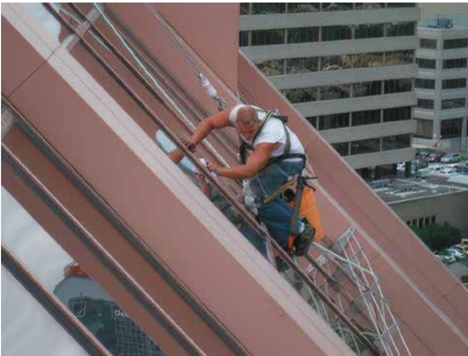
Figure 4. Leak repairs from bosun chair.
