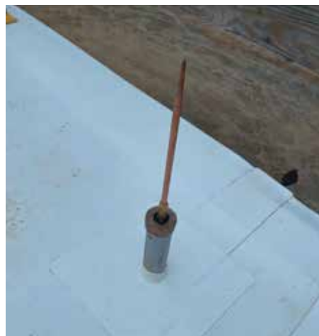
Figure 4. Specialized air terminal design maintains aesthetics while ensuring full lightning protection.
