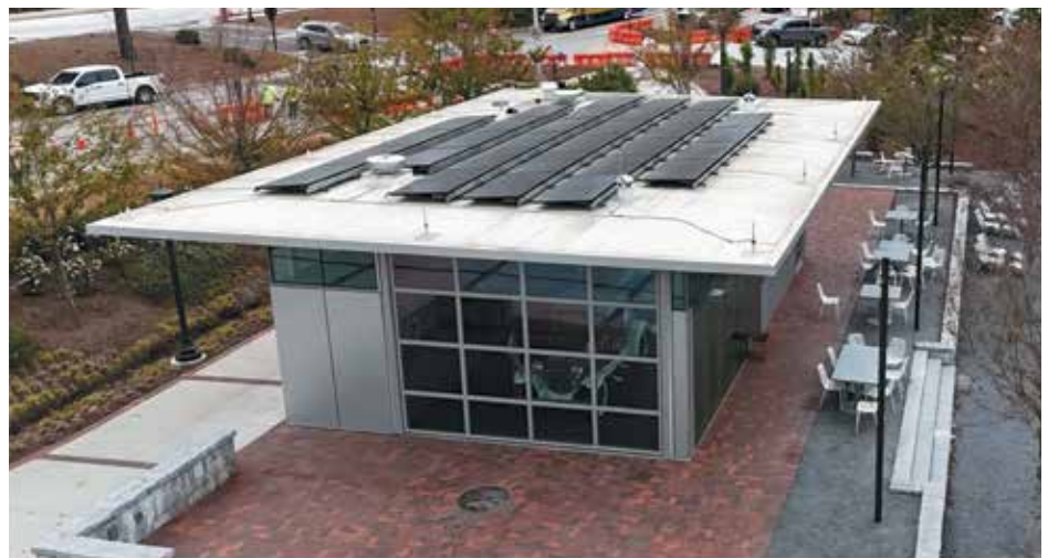
Figure 3. Georgia Tech's net-zero energy garage, home to the iconic Ramblin' Reck. Atlanta Lightning Protection received the Lightning Protection Institute's Most Innovative Design Award for integrating a lightning protection system that preserves both sustainability and tradition. Courtesy of LPI Member, Atlanta Lightning Protection.
