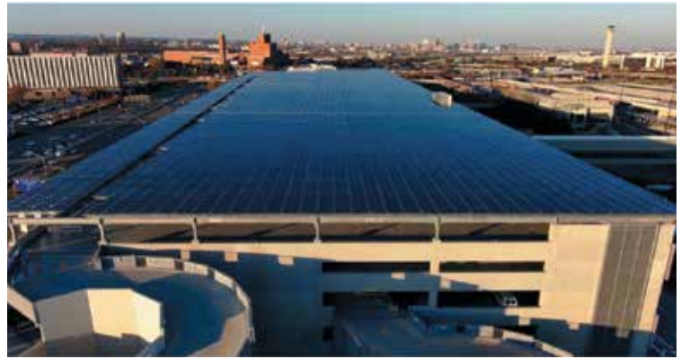
Figure 16. Newark Liberty International Airport's consolidated rent-a-car facility is the largest single solar rooftop project at a US airport and includes a lightning protection system. Courtesy of Lightning Protection Institute member Lightning Prevention Systems.
