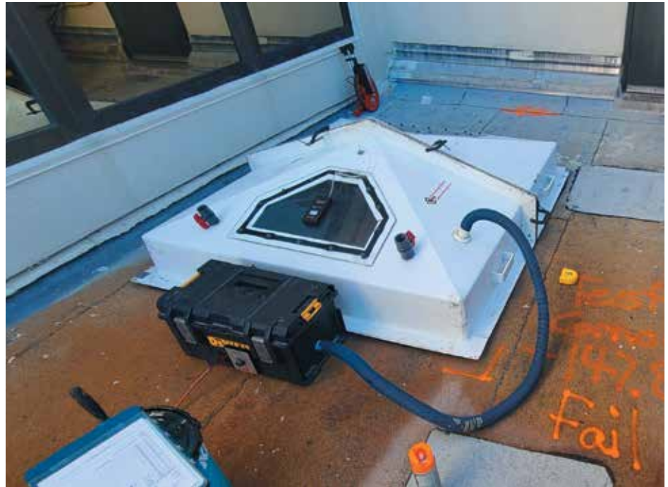
Figure 4. Negative-pressure wind-uplift testing performed over the installed roof system. Several test locations recorded insufficient attachment strength, consistent with membrane plies installed over a damp substrate and asphalt applied at marginal temperatures. This testing confirmed installation-phase deficiencies as the primary failure mode.
