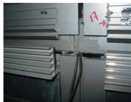
Figure 5. Testing of added heat sinks at a four-way glazing system intersection.
