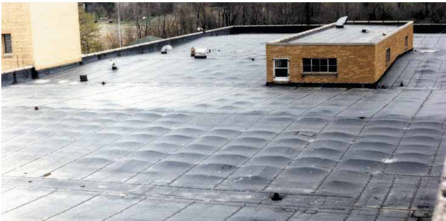
Dimensionally unstable foamed plastic insulation resulted in a failure investigation at this plant in Michigan. Photo courtesy of Roof Engineering Inc.
