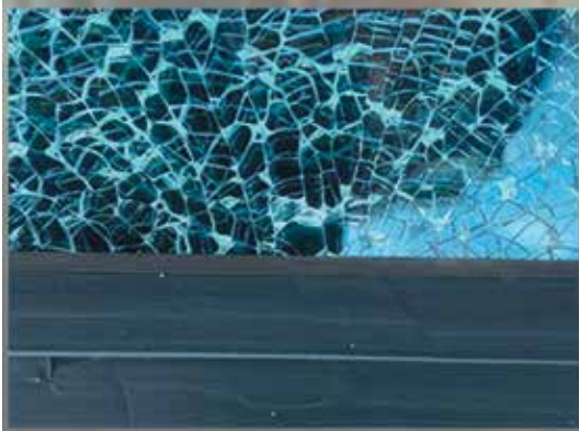
Figure 7. Close-up view of edge glass failure.
