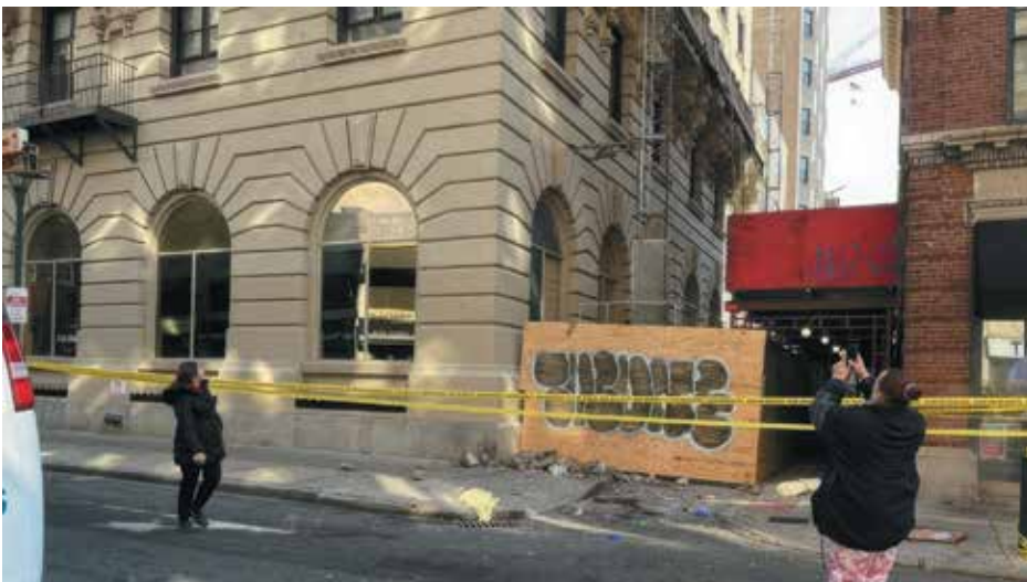
Figure 1. View of 2023 facade collapse debris in Philadelphia's Center City district. Image courtesy of 6ABC. 2
