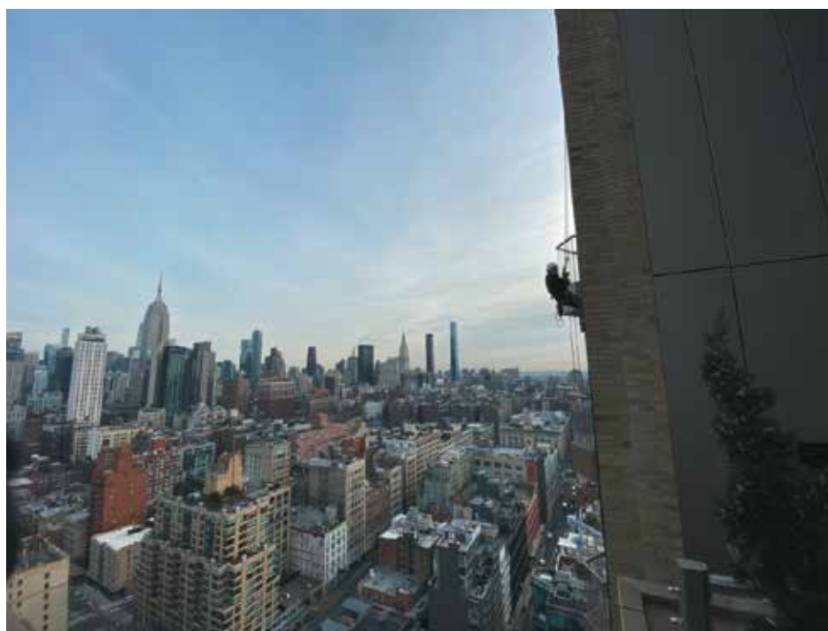
Figure 6. Inspector performing facade inspection via industrial rope access. Photograph by Mike Lopez, January 25, 2022. Rimkus.
