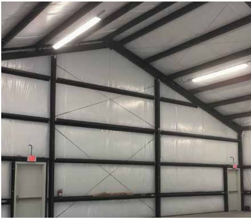
Figure 1. Typical vinyl-faced insulation at the exterior enclosure.
