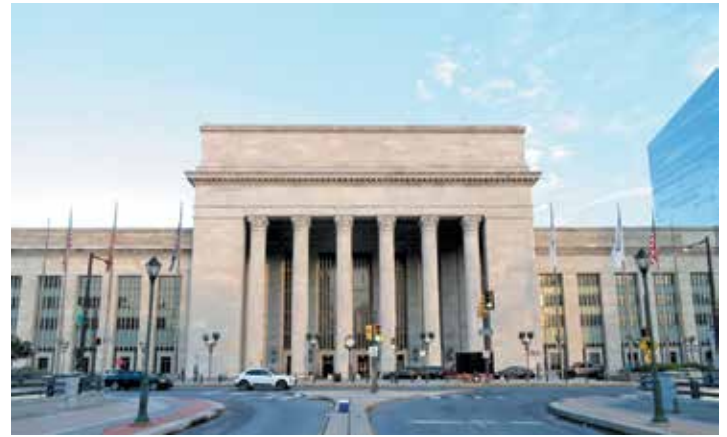
Figure 14. Overall view of completed rehabilitation of the east facade of 30th Street Station in 2018.
