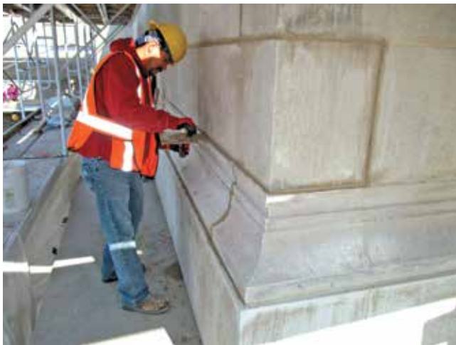
Figure 12. Repointing effort at the limestone at 30th Street Station.
