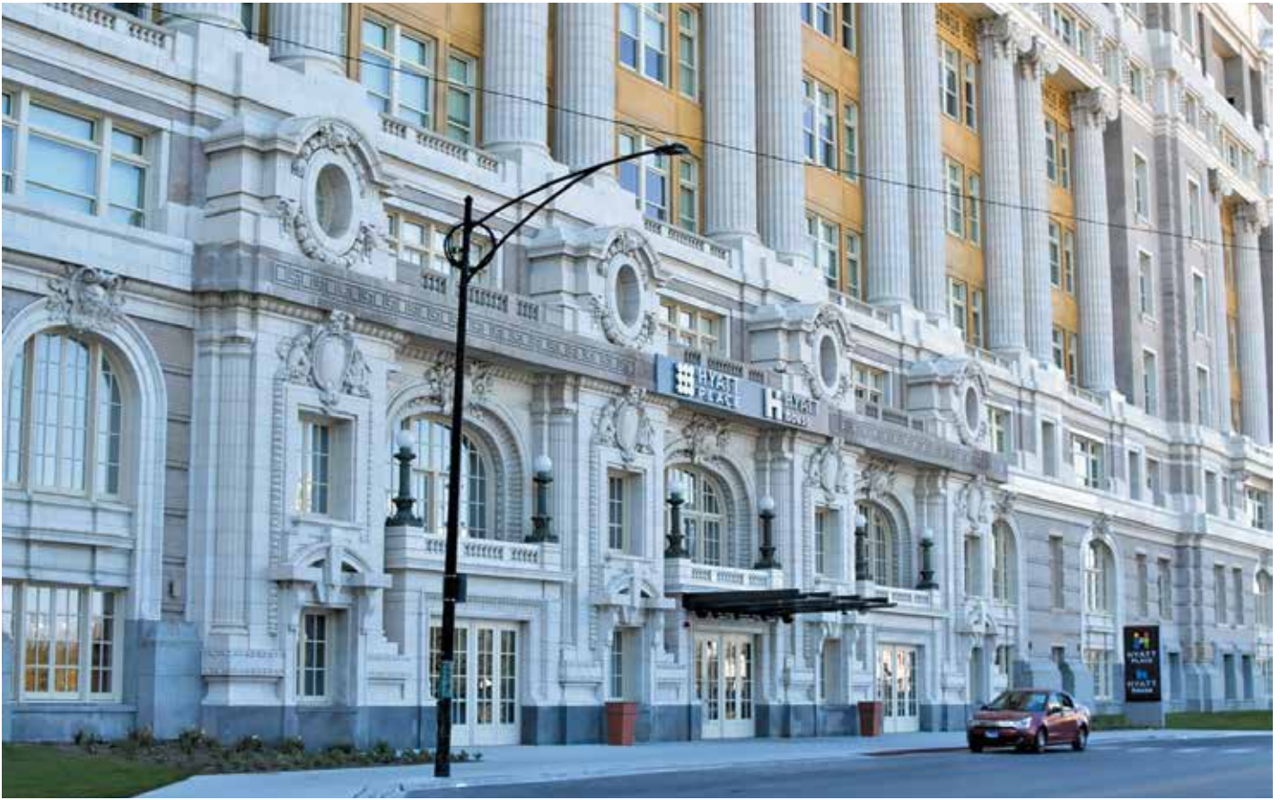
Figure 8. Overall view of the main entrance on the north facade following completion of the Old Cook County Hospital rehabilitation. Note the restored monumental windows and the salvaged and reinstalled the terra-cotta lanterns.
