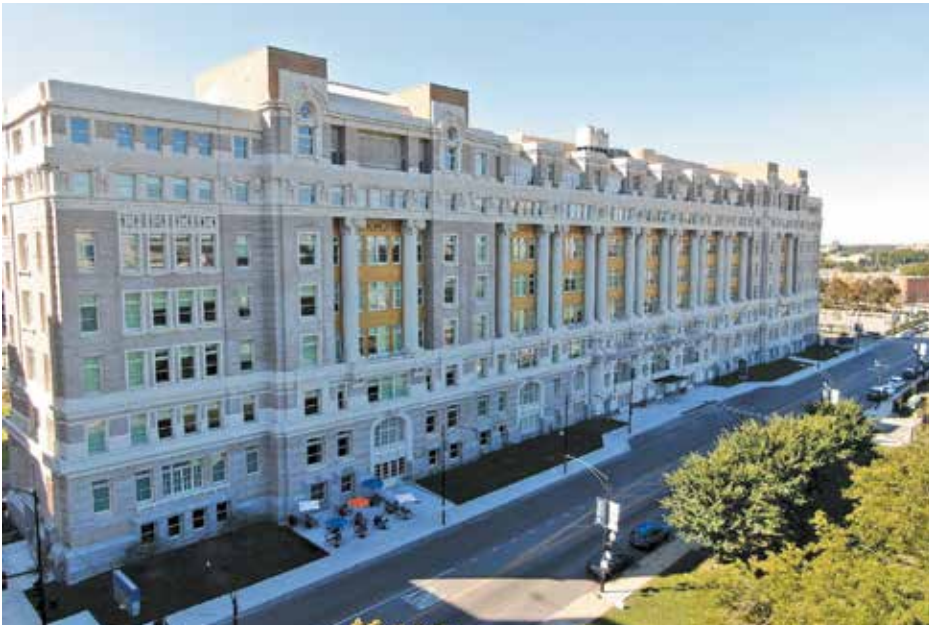
Figure 15. Overall view of completed rehabilitation of the north facade of Old Cook County Hospital in 2020.
