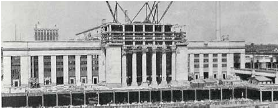
Figure 9. Photo of original construction of 30th Street Station in Philadelphia, Pennsylvania.
