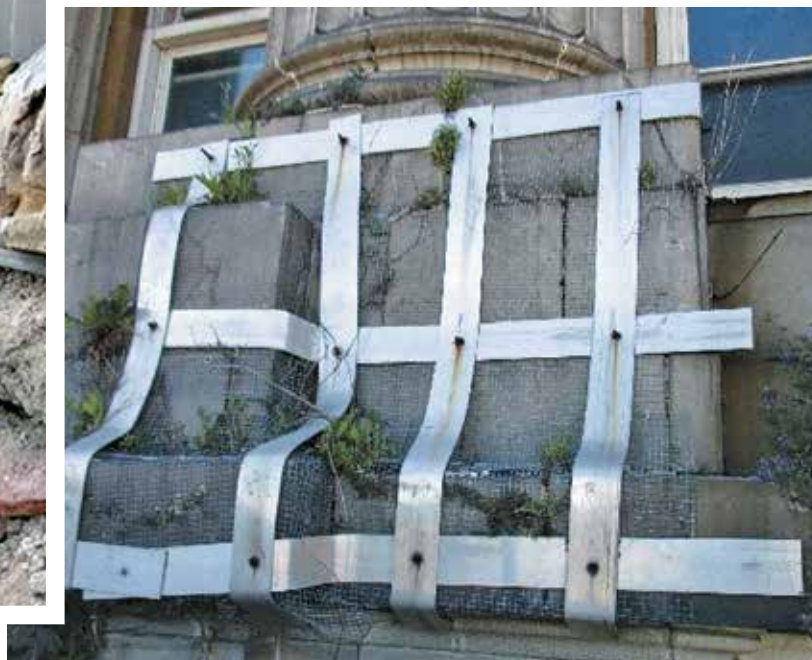
Figure 5. View of distress at the terra-cotta masonry exacerbated by previous stabilization efforts, with corroding fasteners causing cracking and spalling of the terra-cotta units.
