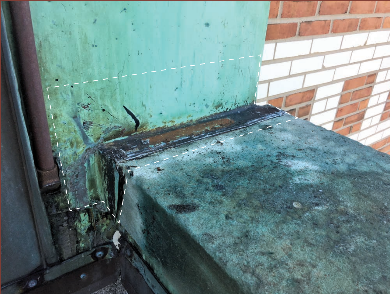
Figure 1. Example of copper saddle flashing (dashed outline) installed on a building constructed in 1913.
