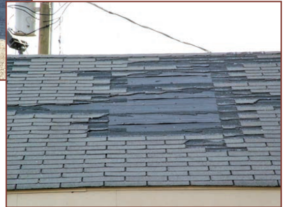
Figure 14. Hurricane Michael. Racking installation.
