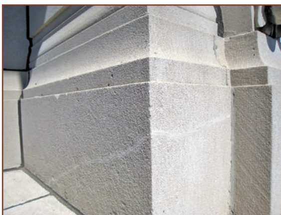
Figure 32. Routed crack pointed with repair mortar.
