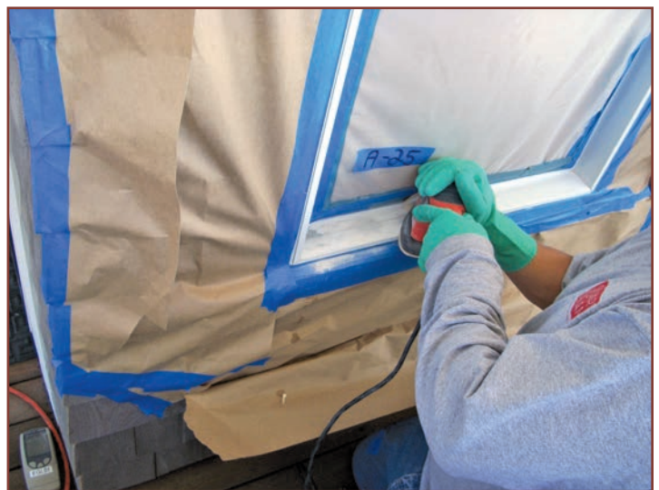
Figure 12. The coating repair process: Sanding down to bare metal. Courtesy of Stuart Dean.
