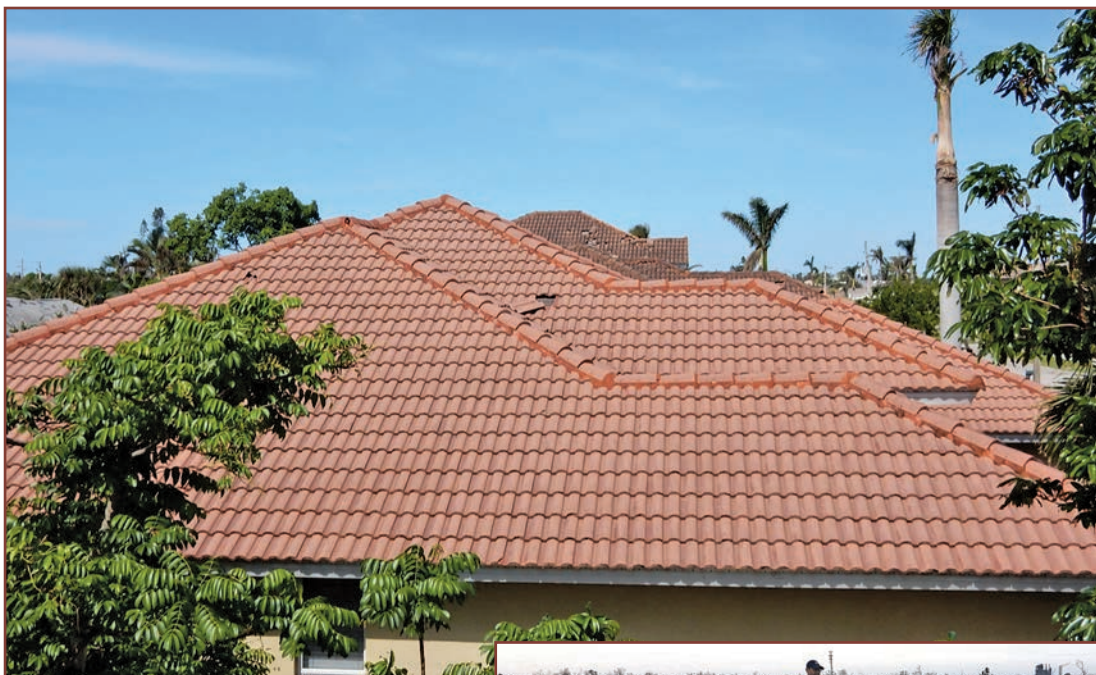
Figure 8. Hurricane Irma: 100 to 100 mph winds. Missile impact damage.
