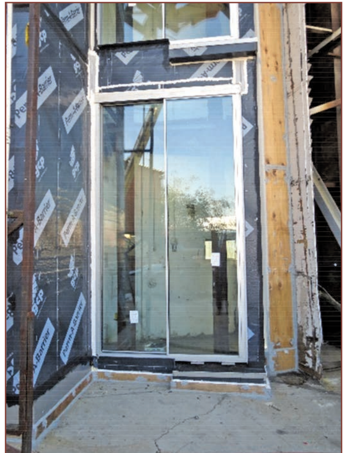
Figure 14. Successfully reinstalled joint installation.
