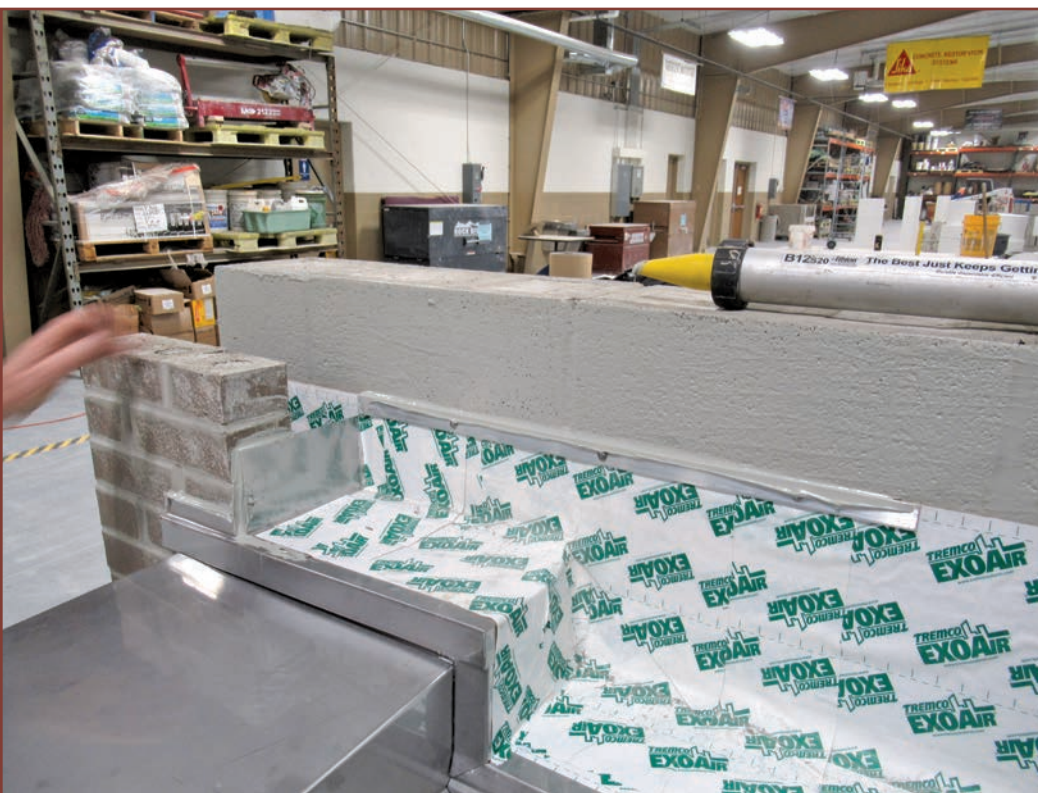
Figure 15. A later stage of the saddle flashing mock-up with all sheet metal components installed and self-adhered flashing membrane in place. The next steps included laying the brick masonry with weeps and installation of a masonry control joint (not shown).
