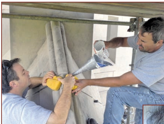
Figure 30. Craftsmen gravity feeding cementitious grout into a cracked joint.
