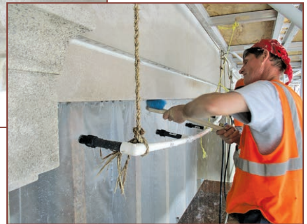
Figure 13. Water misting cleaning at the limestone soffits at the main facades of 30th Street Station.
