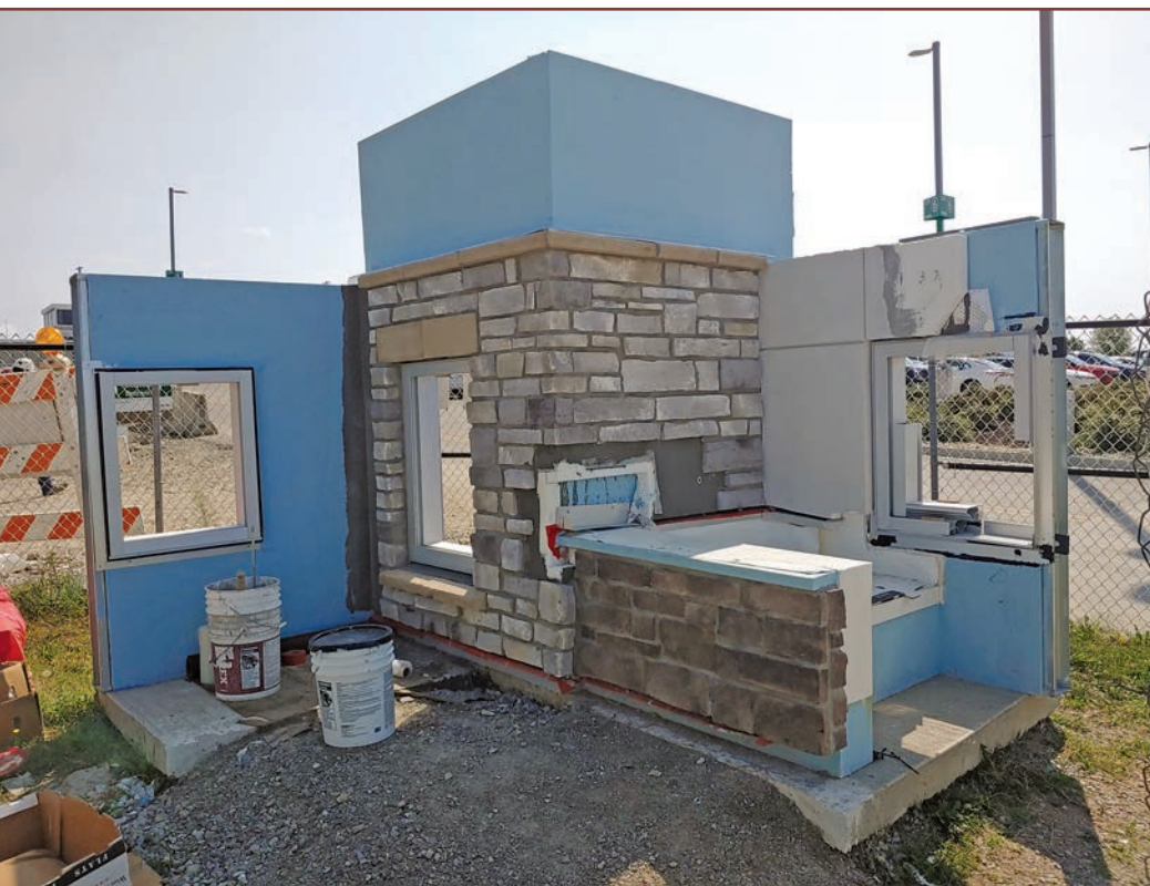
Figure 9. Example of construction mock-up incorporating a saddle flashing condition at the parapet-to-high-rising wall condition. Photograph provided courtesy of M+A Architects of Columbus, Ohio.
