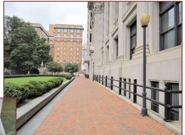
Figure 3. Granite is used as the base course of many limestone buildings.
