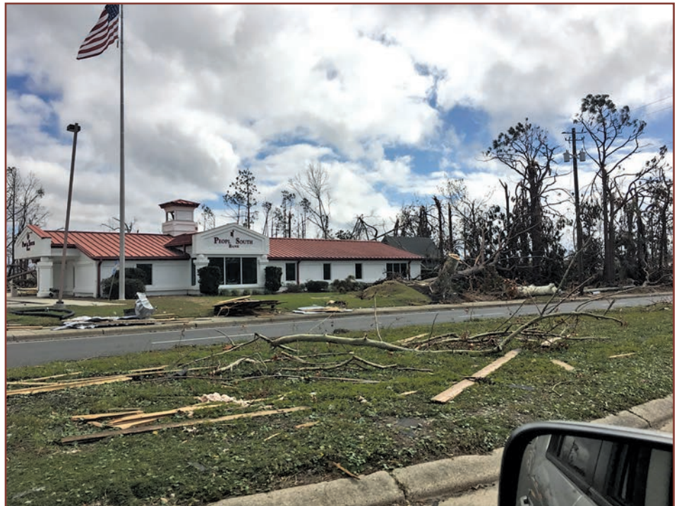
Figure 12. Hurricane Michael: 140 mph winds. The roof on this building, located less than 2 miles from the building shown in Fig. 10, appears to be 100% intact.
