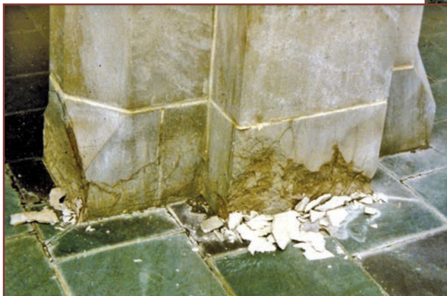
Figure 4. Limestone at grade is prone to freeze/thaw-related deterioration and cryptoflorescence.
