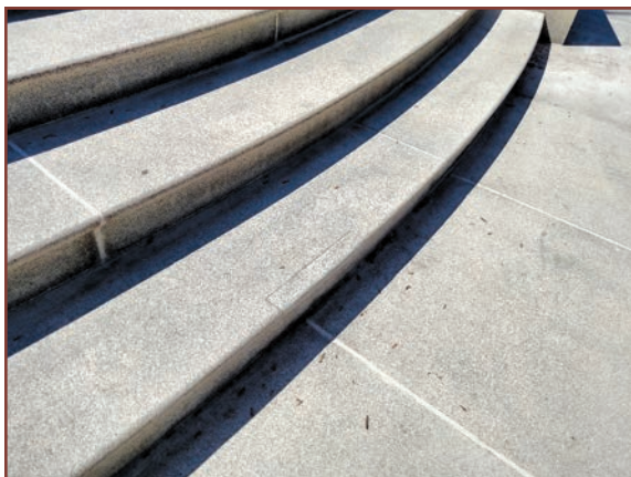
Figure 21. Salvaged granite used as a dutchman, then microabraded to simulate weathering.
