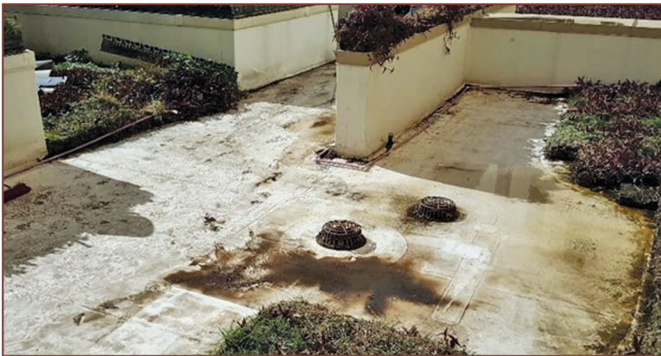
Figure 8. Low-slope roof with vegetative overburden.
