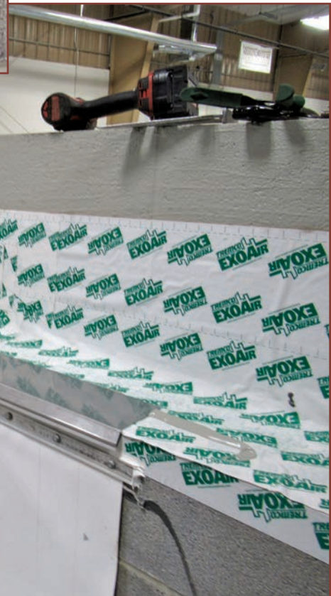
Figure 14. An intermediate stage of the saddle flashing mock-up with the sheet metal saddle, sheet metal drip edge, two-piece counterflashing receiver, and end dam underway.
