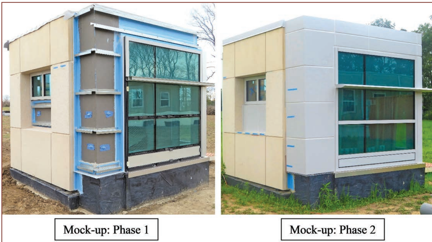
Figure 4. Preconstruction mock-up constructed in two phases.
