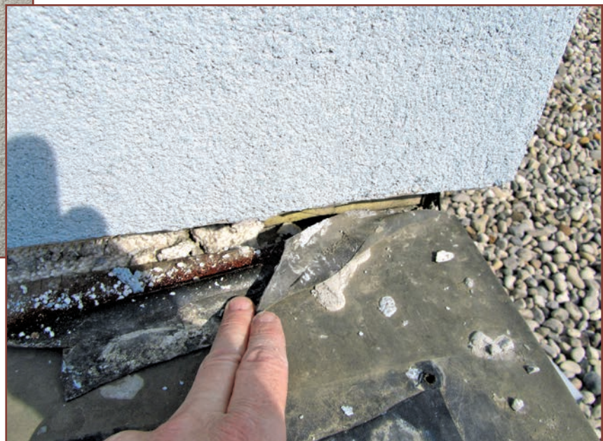
Figure 5. Parapet-to-wall condition with no integration of the single-ply roofing membrane with the exterior insulation and finish systems.
