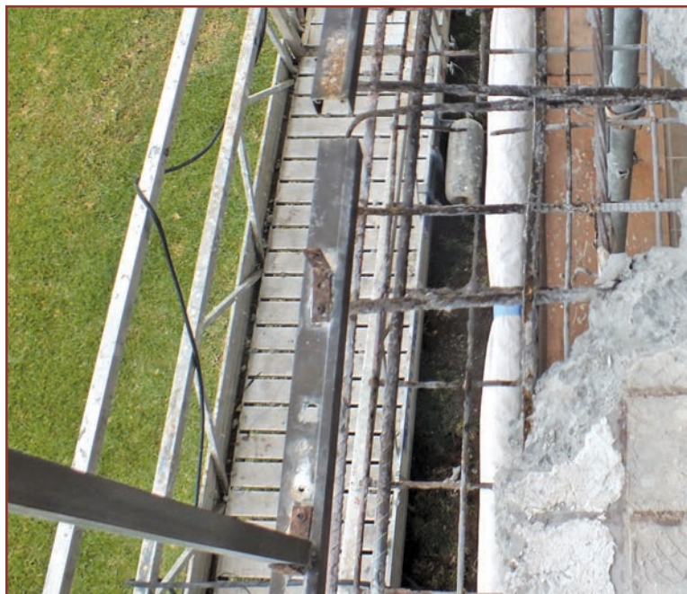
Figure 3. Steel angles used to repair aluminum pickets.
