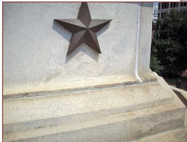
Figure 14. Surface erosion and scaling of granite.
