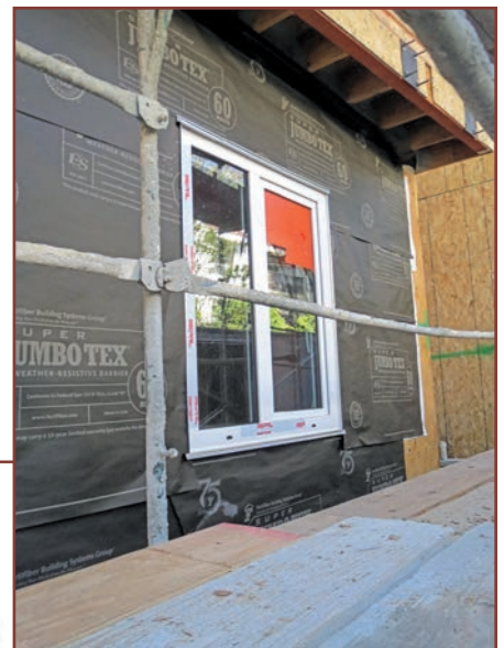
Figure 3. System installation mock-up.
