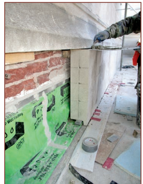
Figure 11. Installation of replacement stone at shelf angle location at 30th Street Station.
