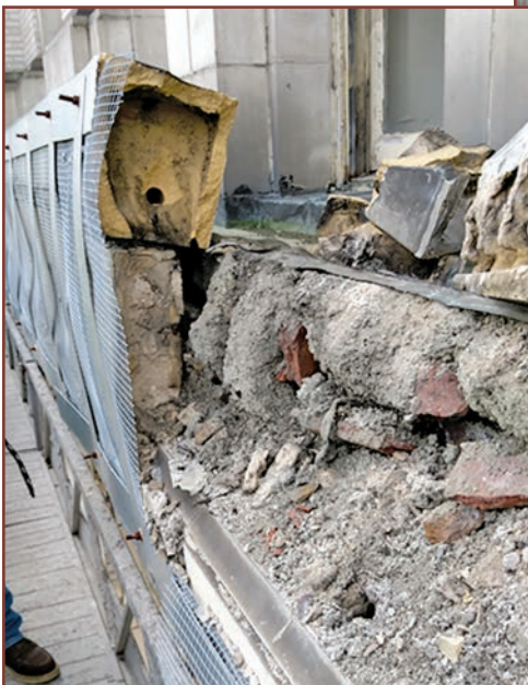
Figure 5. View of distress at the terra-cotta masonry exacerbated by previous stabilization efforts with corroding fasteners causing cracking and spalling of the terra-cotta units.
