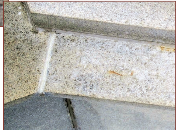
Figure 35. Sealant installed at a skyward-facing joint. Note that the mortar is installed in the joint below.
