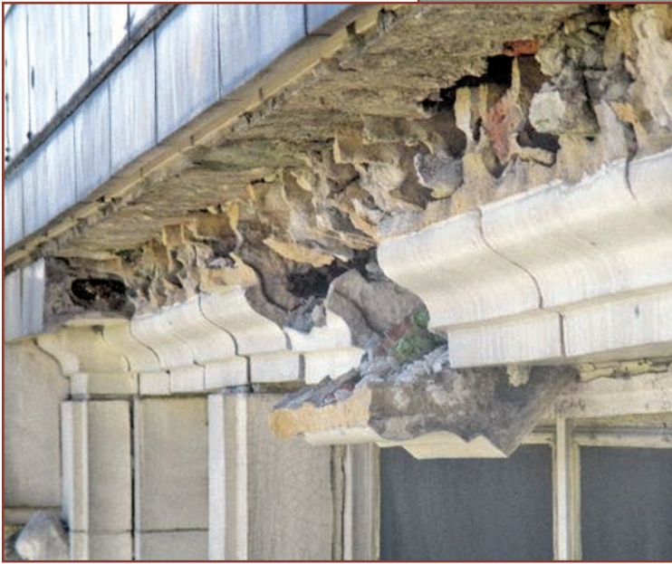
Figure 4. Distressed terra-cotta window seventh floor head units below previously replaced cornice caused by corrosion of steel anchorages poor detailing of retrofit at Old Cook County Hospital as viewed during 2016 Phase 2 assessment.
