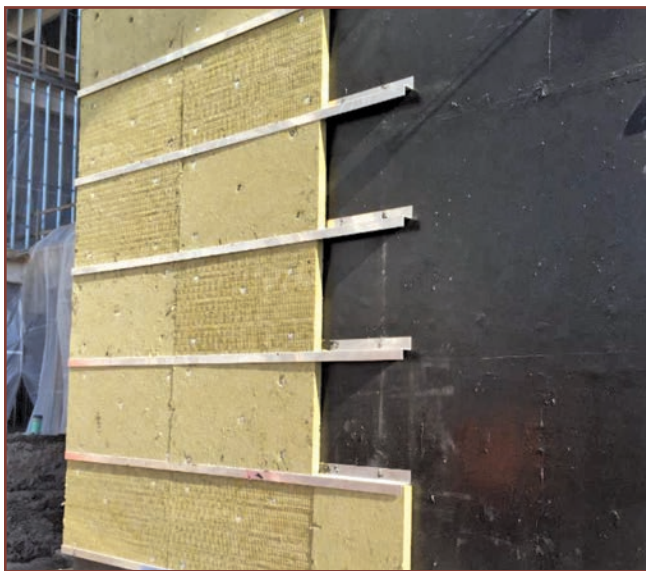
Figure 1. Photograph of exterior insulation with continuous metal Z girts installed through insulation.
