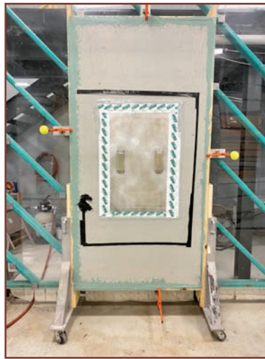
Figure 3. Mock-up 1, round 2 testing, fluid-applied WRB system. Note: WRB = water-resistive barrier.
