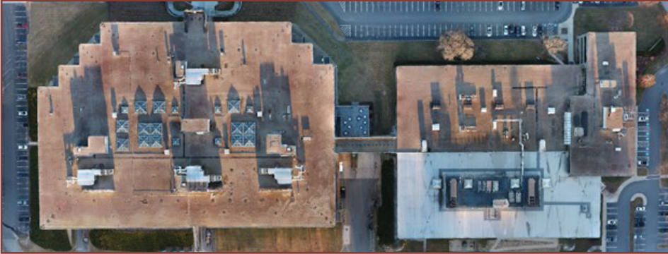
Figure 9. Fully stitched digital image of the roof.
