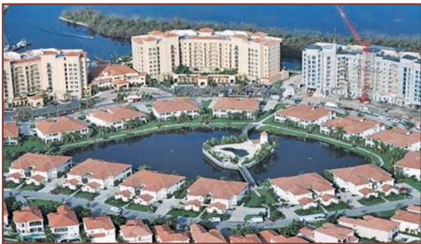
Figure 4. Hurricane Charley: Likely 130 to 140 mph winds. New units, foam adhesive. Very minor damage.
