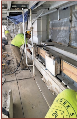
Figure 7. Reconstruction of the third floor gutter and installation of terra-cotta units at the north, east, and west facade during rehabilitation in 2018–2019.
