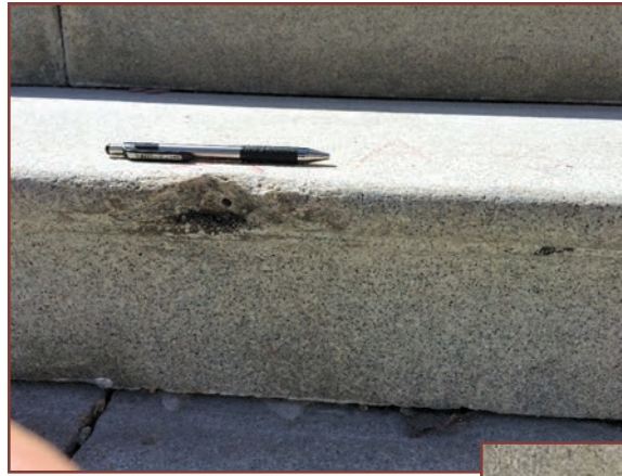
Figure 18. Small spill on a stone tread; no consequential damage is likely if left unrepaired.
