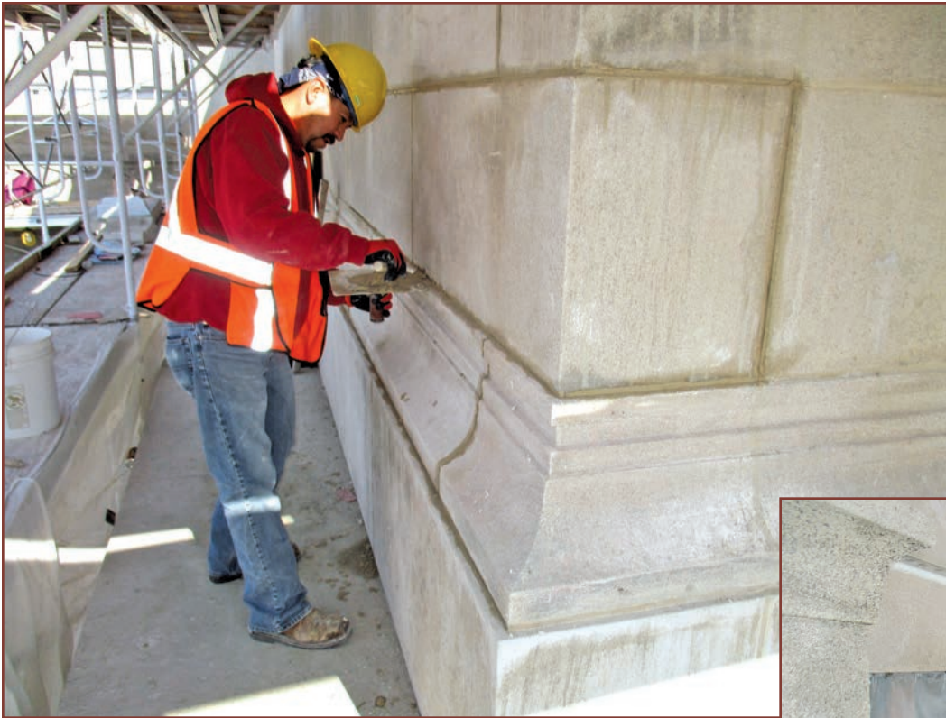
Figure 12. Repointing effort at the limestone at the 30th Street Station.
