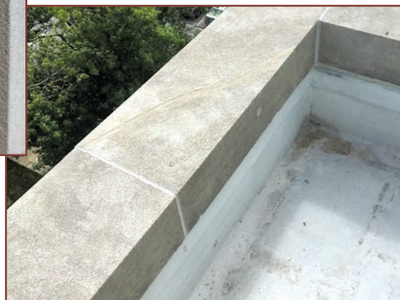
Figure 33. Routed crack filled with sealant.
