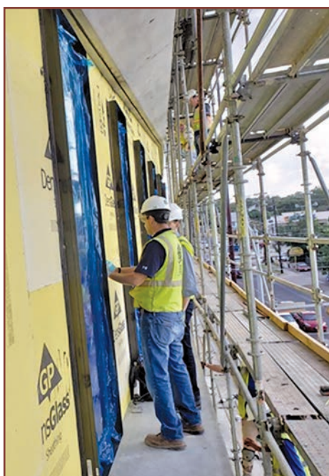
Figure 13. Commercial flanged window installation.
