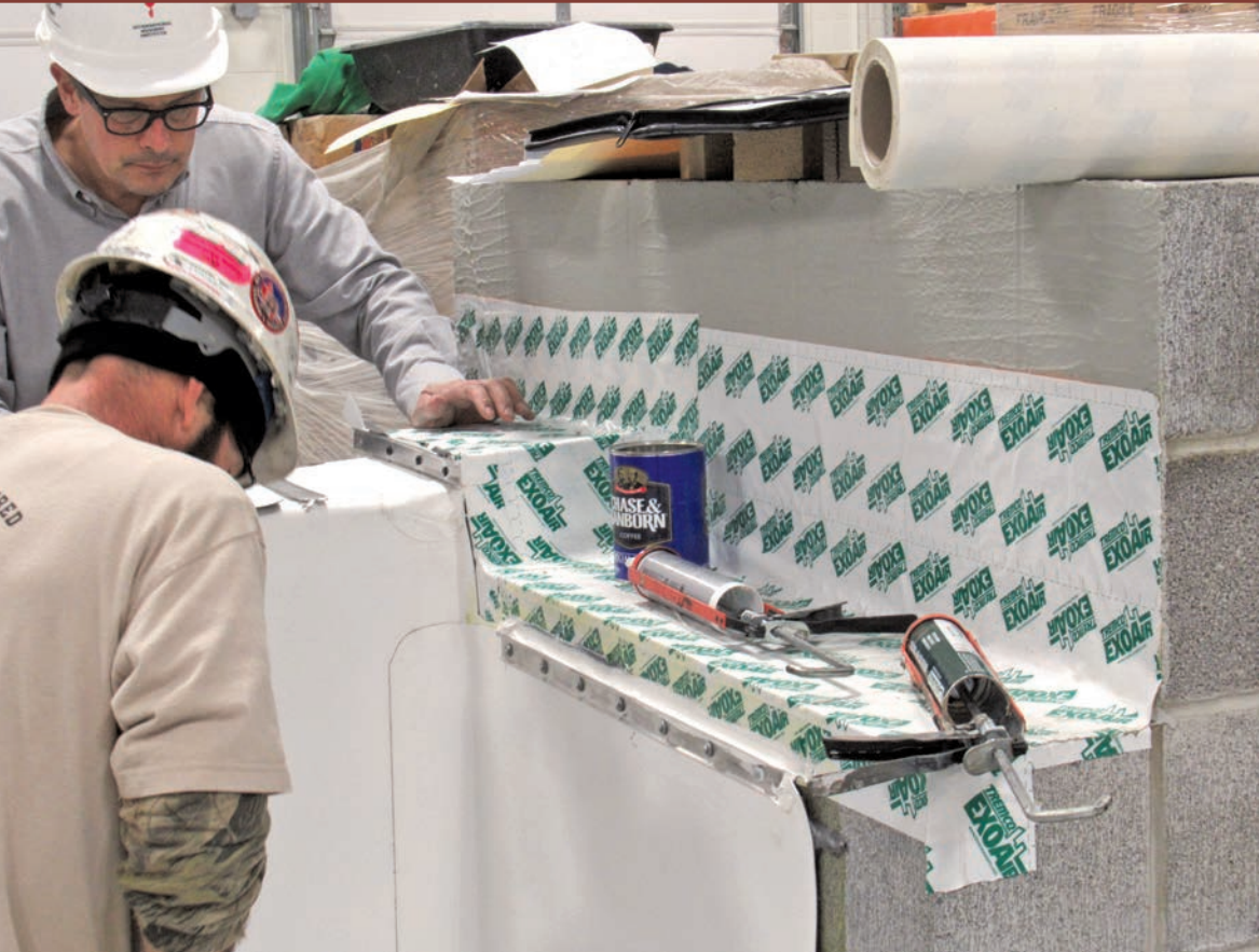
Figure 13. An early stage of the saddle flashing mock-up before the installation of the sheet metal through-wall flashing, saddle flashing, and coping.
