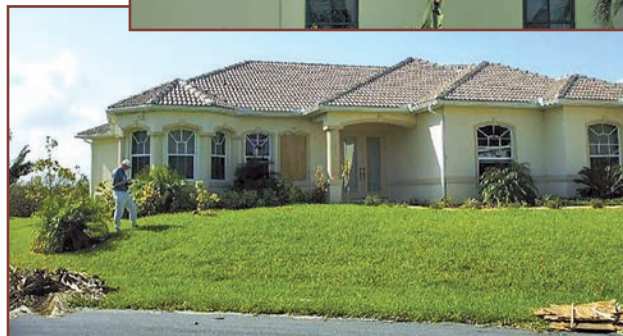
Figure 3. Hurricane Charley: 130 mph winds. Ridge damage on this roof.
