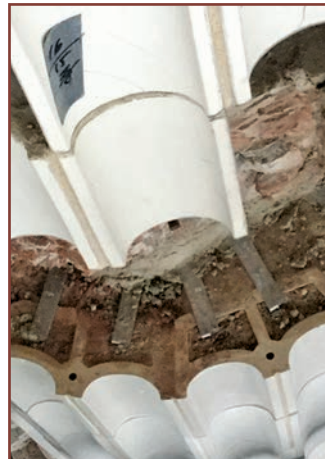
Figure 6. Installation of terra-cotta units at monumental columns at the north facade during rehabilitation in 2019.
