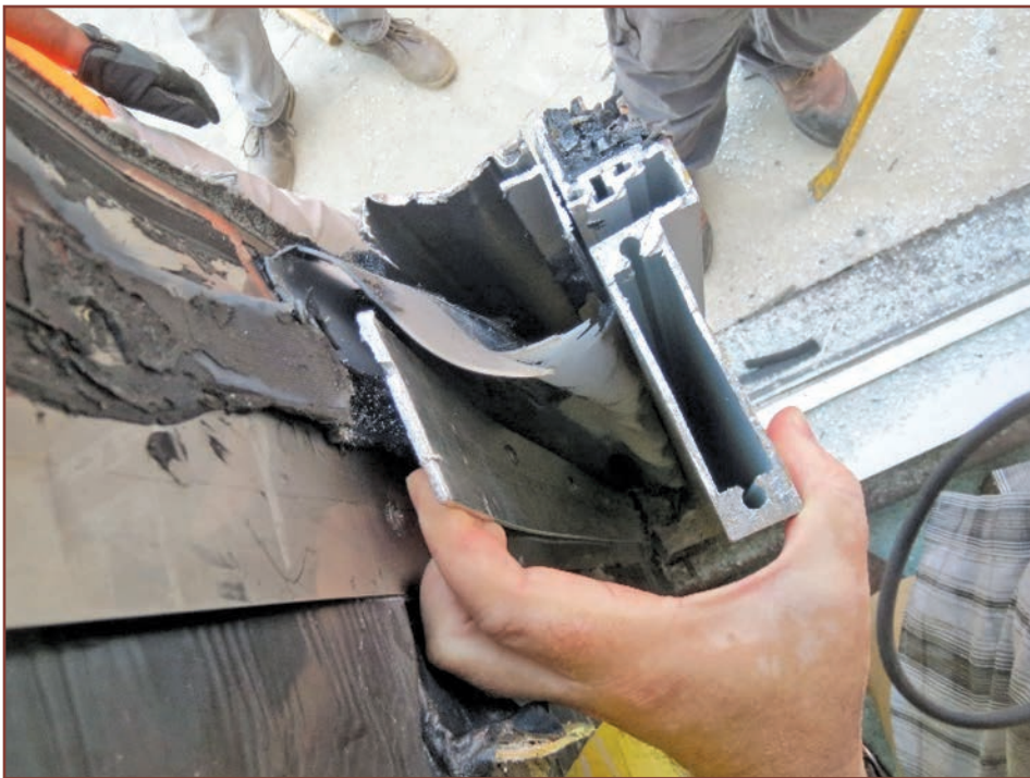
Figure 15. Deconstruction of performance mock-up components.
