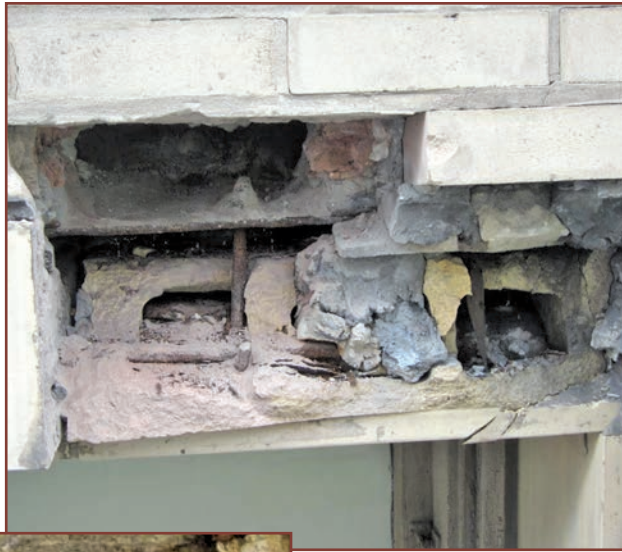
Figure 3. Distressed terra-cotta window head unit caused by corrosion of steel anchorages and support at Old Cook County Hospital as viewed during 2011 Phase 1 assessment.
