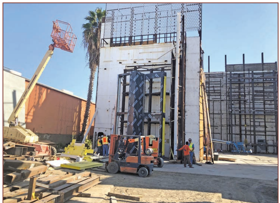
Figure 9. Performance mock-up in construction.
