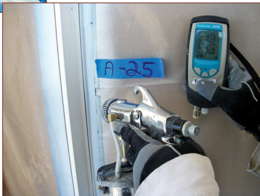
Figure 14. The coating repair process: Top coat application. Courtesy of Stuart Dean.
