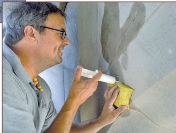
Figure 31. Craftsman injecting resin grout into a crack.
