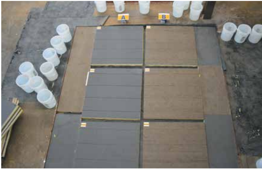
Figure 1. Lines were drawn on the insulation boards (with spacings centered on boards) to guide the application of the low-rise foam adhesive ribbons. The lines were centered so that application of the adhesive would be symmetrical. The photo shows the line layout for a 12 in. ribbon spacing.
