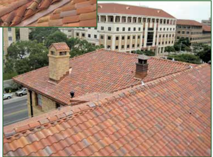
Littlefield Dormitory showing tile and copper flashings.
