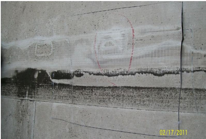
Figure 2 – Embrittlement of thermoplastic membrane from self-adhesive, bituminous-based flashing.
