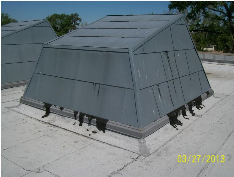
Figure 1 – Black flow from self-adhesive, bituminous-based flashing.
