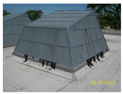
Figure 1 – Black flow from self-adhesive, bituminous-based flashing.
