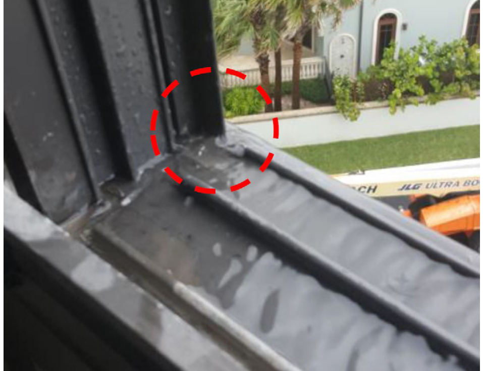
FIGURE 1. Base of Sliding Window was previously blocked and allowed water accumulation.
