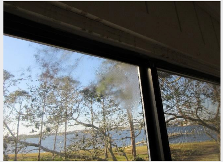
FIGURE 10. Typical window damage (fogged lite).
