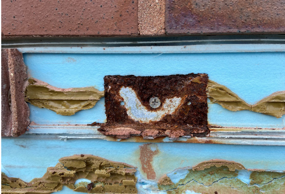
FIGURE 2. Insulation clip in the wet zone of the wall, which has begun to corrode.
