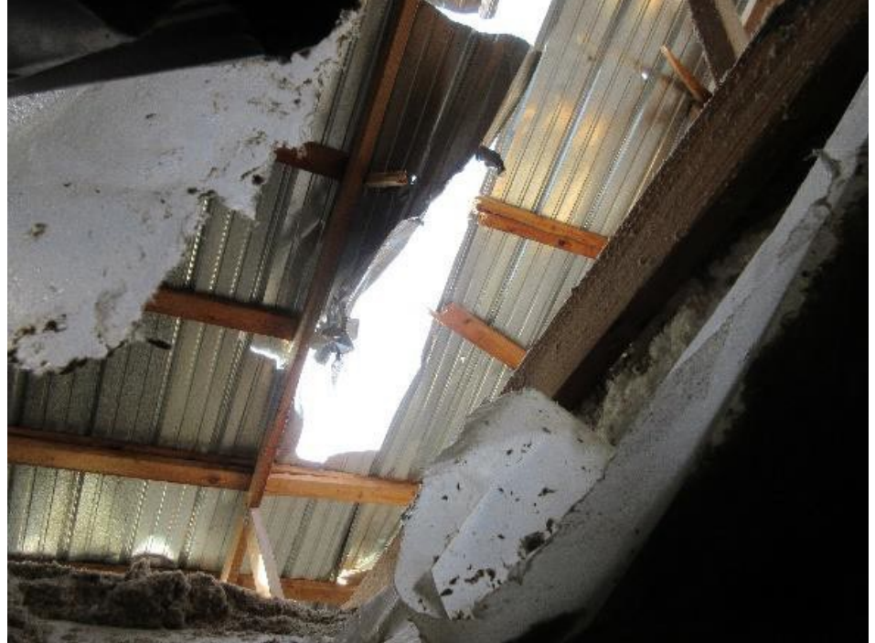
FIGURE 2. Dangerous roof condition with broken and dangling roof members and cladding.
