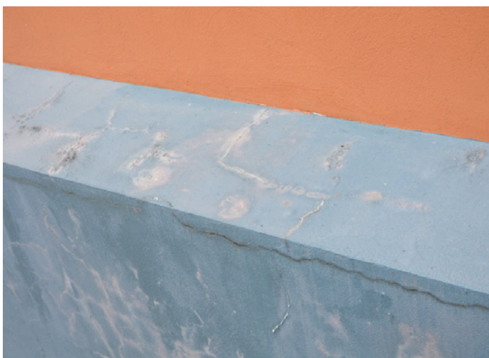
FIGURE 9. Stucco on water table is cracked.
