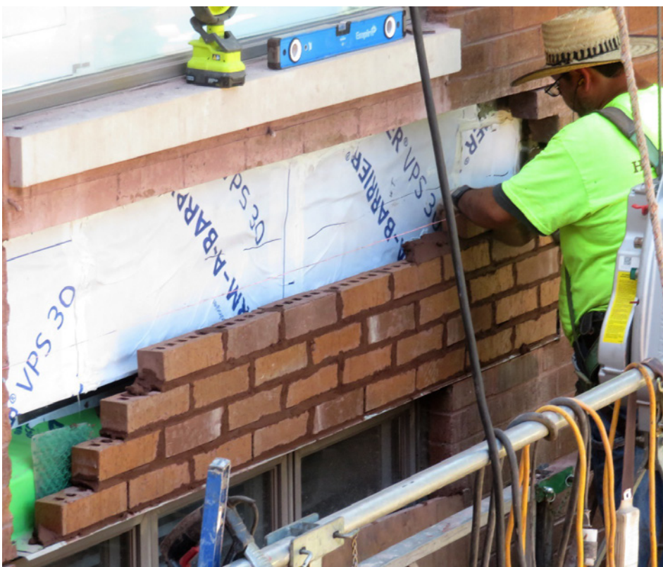
FIGURE 10. Installation of brick veneer following installation of the AWB and through-wall flashing.
