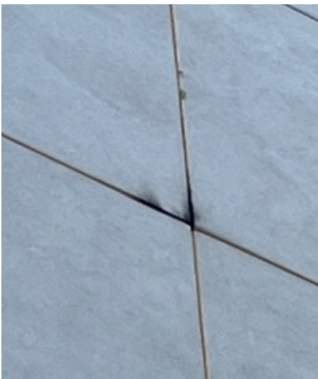
FIGURE 9. Weld damage on the exposed exterior face of a prefabricated panel.
