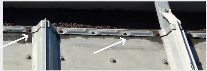
FIGURE 12. Representative panel eave location being last to dry after rain or morning dew.
