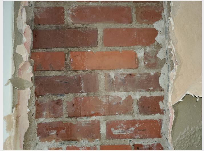
FIGURE 7. Representative view of damp portion of wall with water weeping from anomalies at the interior masonry surface.
