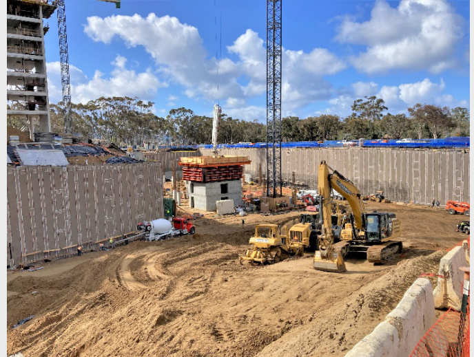
FIGURE 1. Waterproofing at a deep foundations site.
