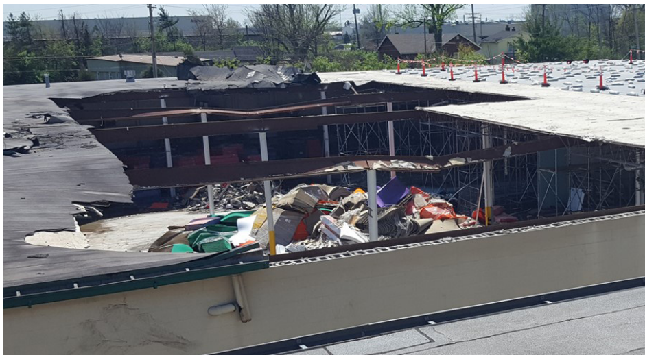
FIGURE 3. Warehouse failure. (Source: Carlisle Construction Materials)
