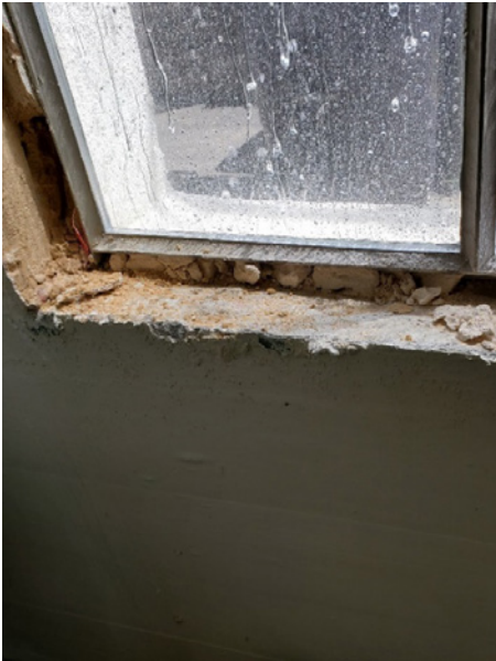
FIGURE 14. Representative view of soft stucco wrapped into the window rough opening.
