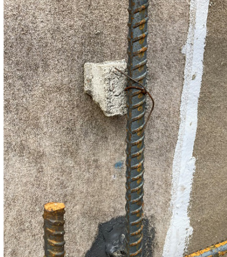
FIGURE 6. Dobie block placed between rebar and waterproofing membrane.
