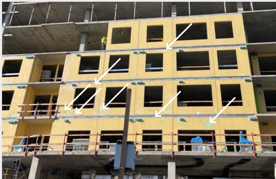
FIGURE 6. Panels with damaged AWB membrane from stacking during transport.
