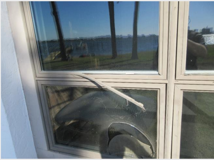
FIGURE 9. Typical window damage (broken lite and displaced glazing bead).
