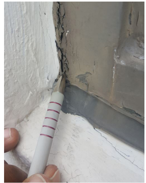
FIGURE 2. Aged sealant conditions around a window.
