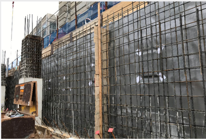
FIGURE 2. Pre-applied blindside waterproofing installed prior to pouring of concrete wall.
