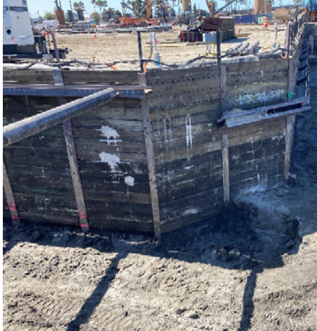
FIGURE 4. Example of front-lagged lagging wall.
