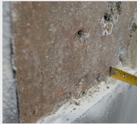
FIGURE 7. Stucco thickness was measured to be approximately 1 inch thick.
