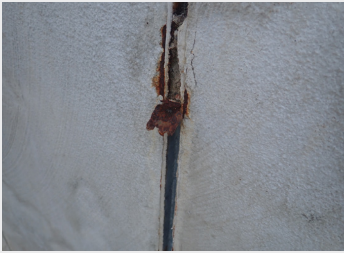
FIGURE 9. Corroded galvanized brick tie.
