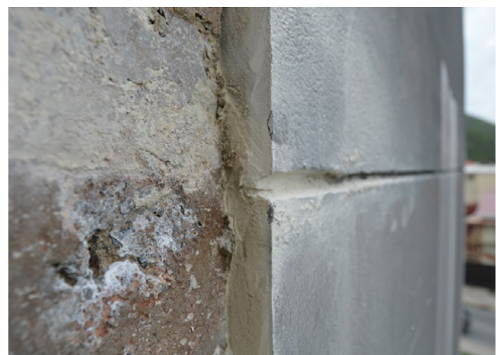
FIGURE 10. Destructive opening at a reveal of the stucco. No joint accessories were observed.
