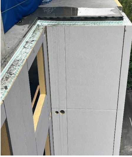
FIGURE 8. Stains from ponded water running off temporary waterproofing and over panel finished surface
