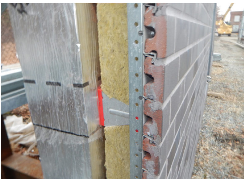
FIGURE 4. Thin brick rail system on a rainscreen support system.
