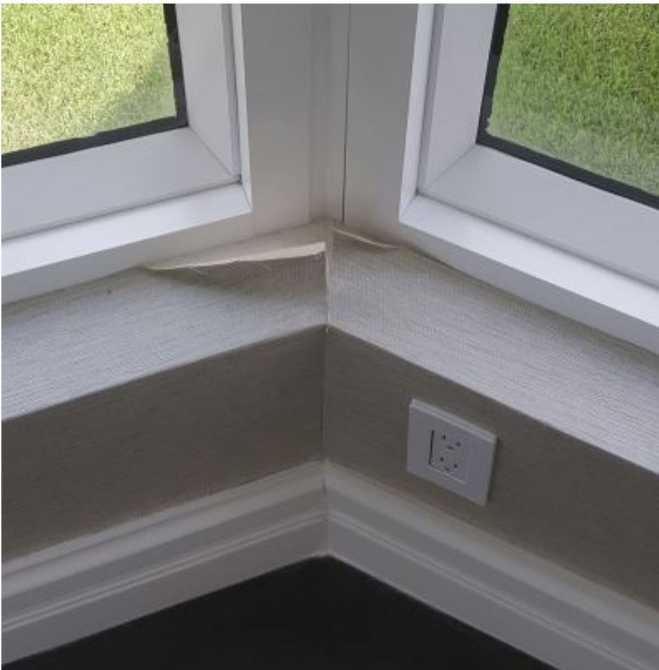
FIGURE 6. Distortion at window.
