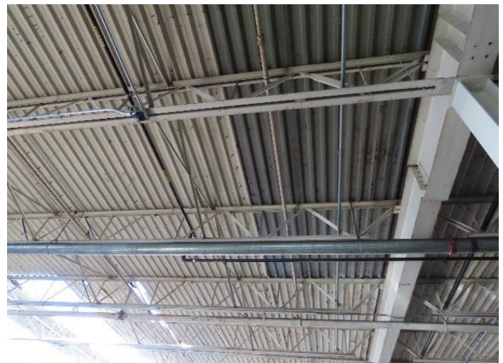
FIGURE 6. Replacement deck at right center.
