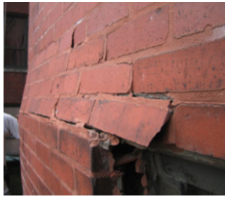
FIGURE 7. Displaced masonry due to corroded lintel.
