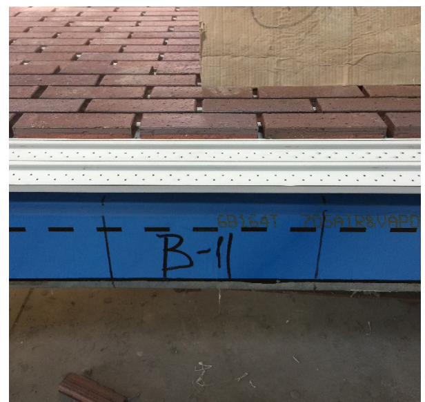
FIGURE 5. Panelized thin brick rail system project during construction, rails installed, bricks set in place, mortar work not yet complete.
