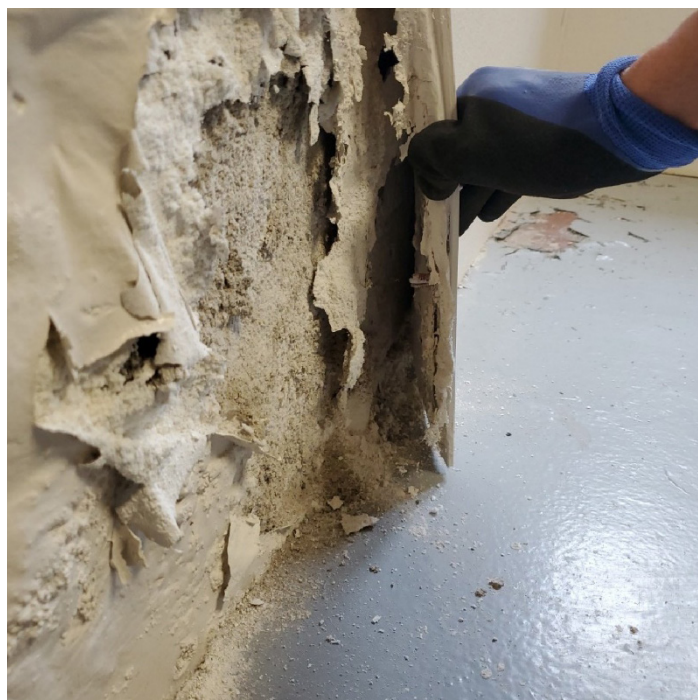
FIGURE 3. View of low permeability barrier installed at wall interior.
