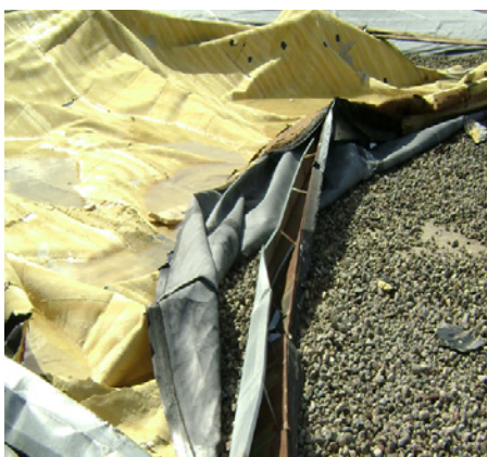
FIGURE 6. Gutter securement failure. (Source: Carlisle Construction Materials)
