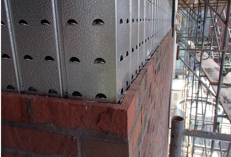
FIGURE 1. Panel-mounted, proprietary TBV with formed corner tiles.
