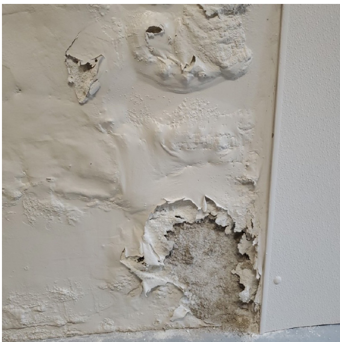
FIGURE 2. View of moisture-related damage to interior finishes.
