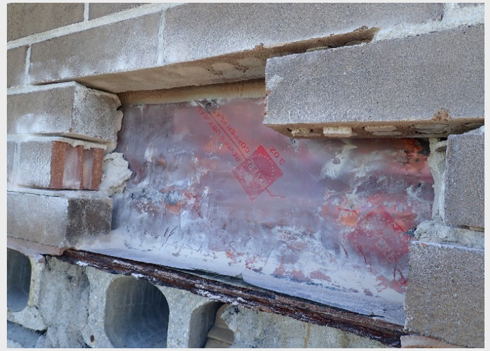
FIGURE 10. View of shelf angle detailing.
