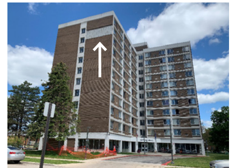
FIGURE 8. Overview of failure. Note large area on facade with missing masonry cladding.
