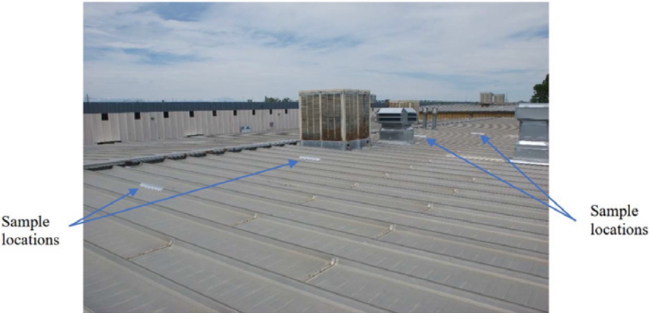
FIGURE 3. The 55%Al-Zn alloy-coated steel SSR with sample locations.
