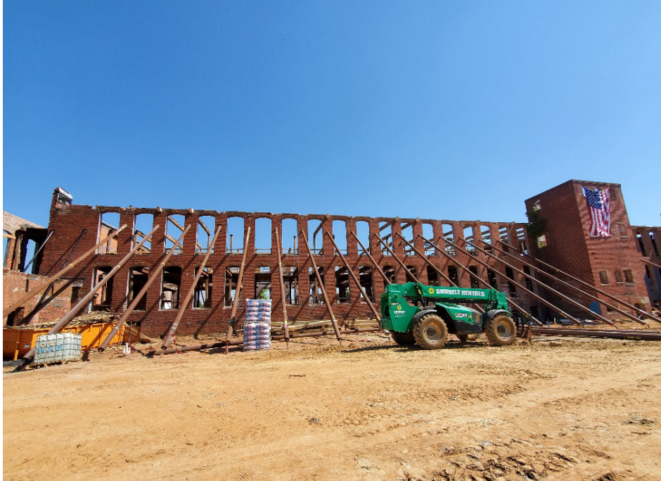
FIGURE 1. Overview of previous industrial mass masonry structure during construction of adaptive reuse project.
