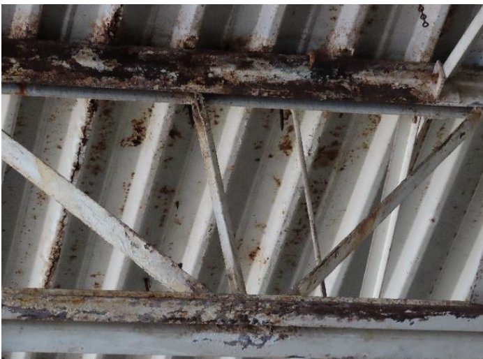
FIGURE 5. Typical metal deck corrosion.
