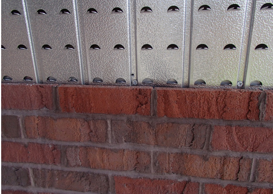
FIGURE 3. Panel-backed TBV system.
