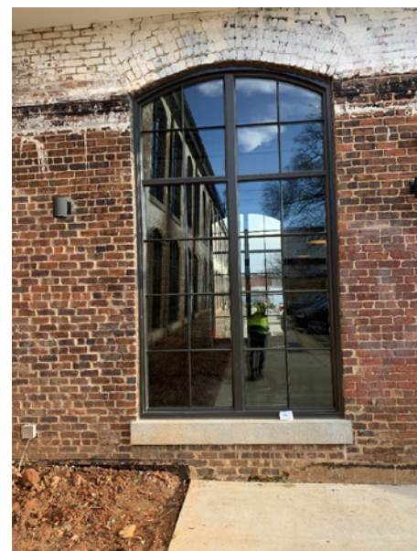
FIGURE 10. Representative view of new fenestration installed in existing mass masonry wall opening.
