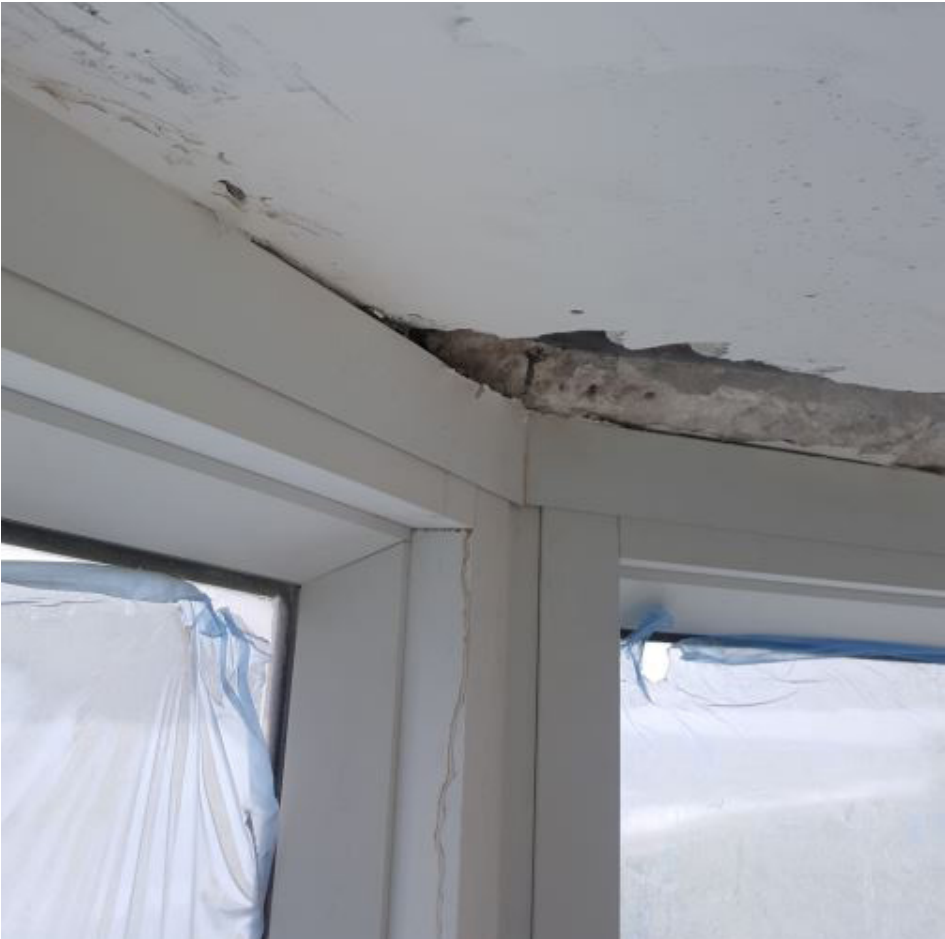
FIGURE 4. Red stains reveal compromised conduit not window assembly.
