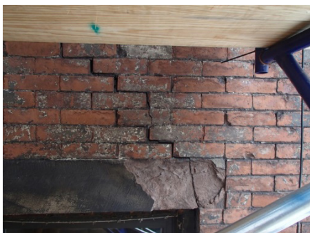
FIGURE 6. Step cracking due to corroded lintel.
