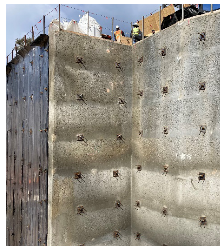
FIGURE 5. Soil nail wall with exposed nail heads and bearing plates.
