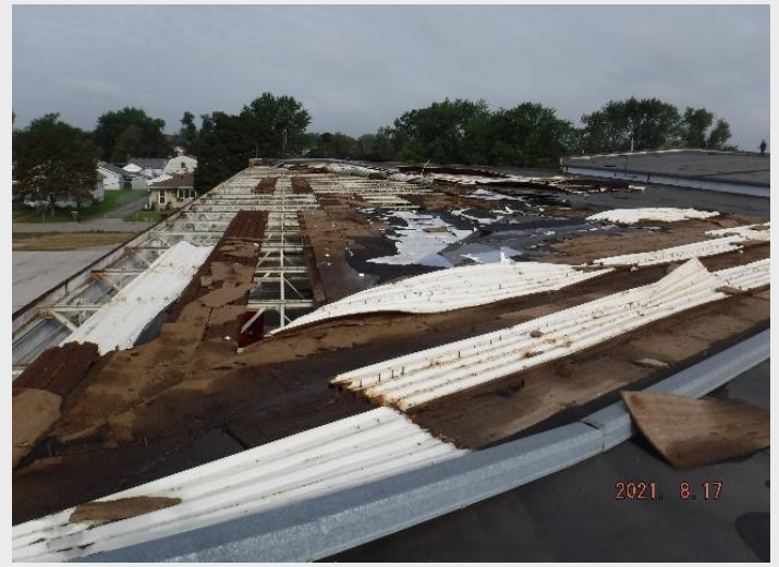
FIGURE 4. Wind damage in the southwest corner of the roof.
