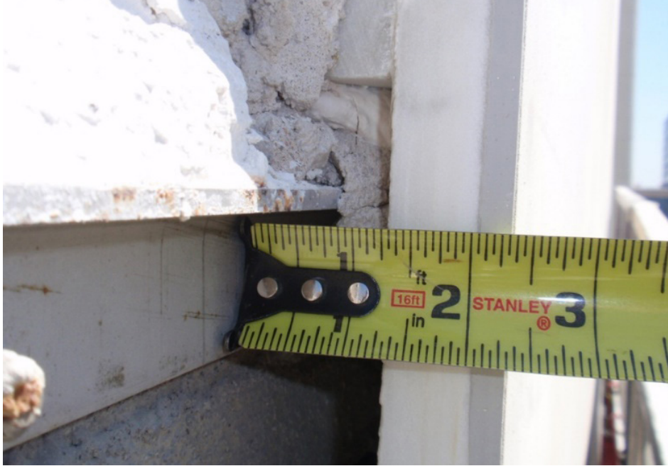
FIGURE 15. Gravity support of panels consisting of a liner block adhered to the back of the panels and bearing on a shelf angle.
