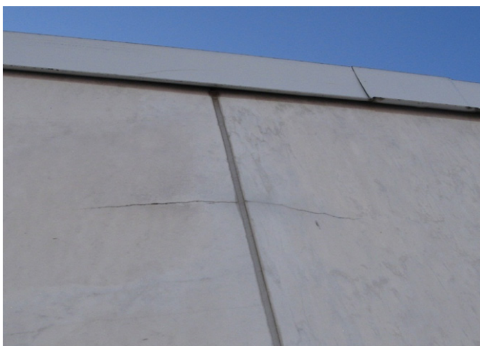
FIGURE 13. View of typical cracking of panels.
