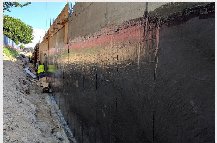
FIGURE 3. Installation of post-applied waterproofing membrane.
