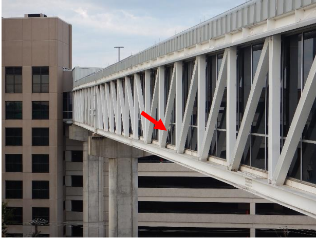
Figure 38. Broken spandrel lite on east facade above rail road track.
