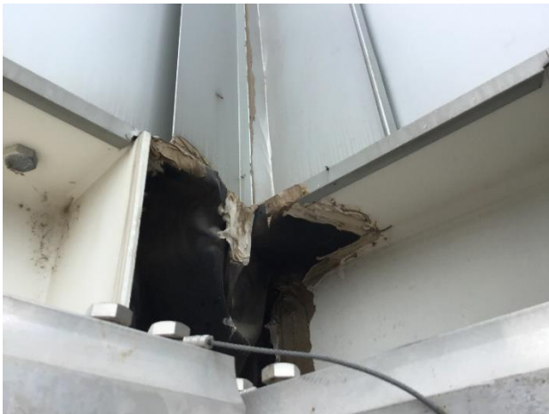
Figure 14. Black flexible membrane at steel beam intersection for Skybridges A and B.
