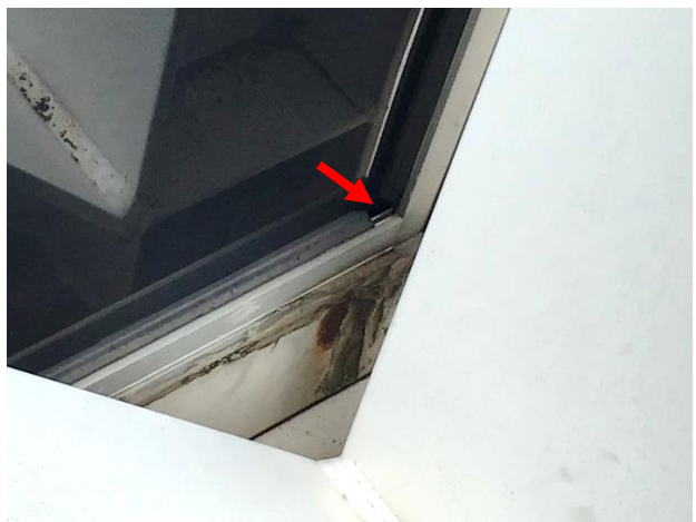
Figure 7. Gasket shrinkage at sill of window wall.
