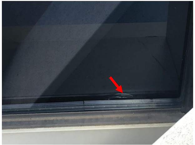
Figure 41. Deficiency observed within perimeter IGU seal.
