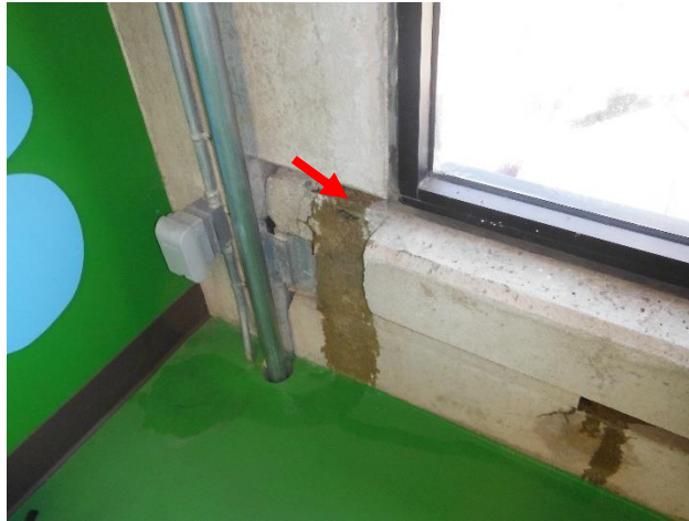
Figure 73. Immediate water intrusion observed due to large discontinuity in perimeter sealant at the corner of the window.
