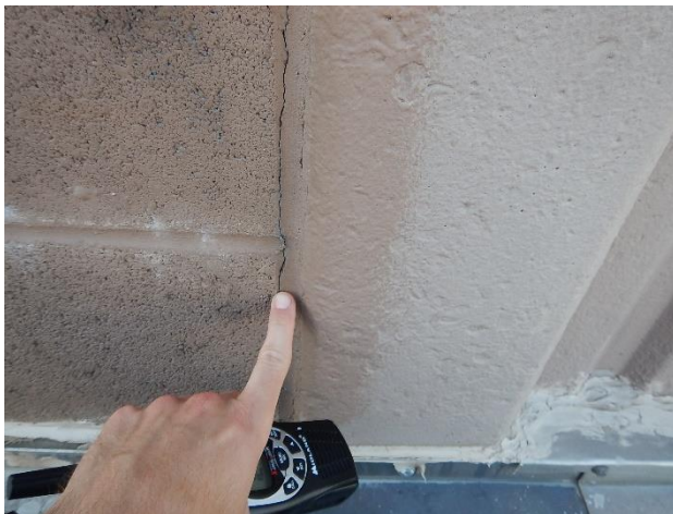
Figure 62. Separation/cracking of mortar joint within CMU infill above roof flashing.
