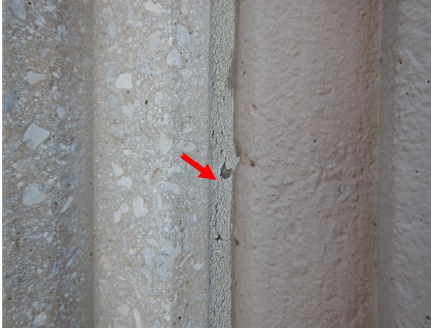
Figure 64. Cohesive failures of precast-to-precast sealant joint.
