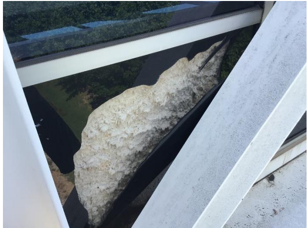
Figure 39. Broken spandrel lite on east facade above rail road track.
