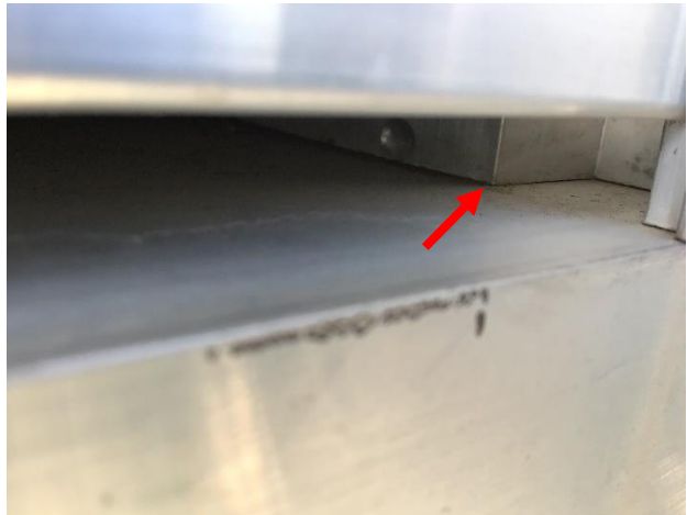
Figure 33. Open joint observed inside louver.
