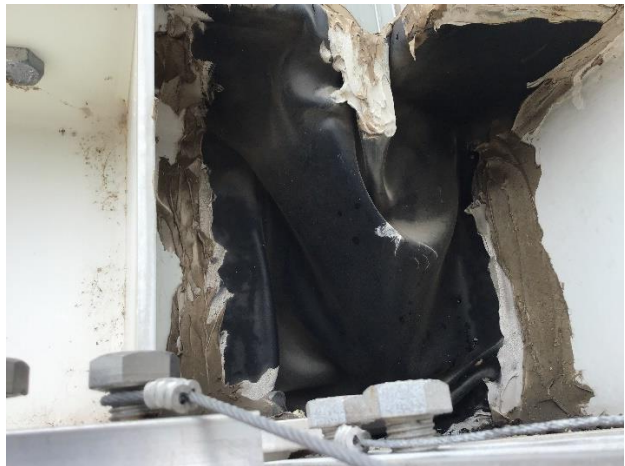
Figure 15. Two different applications of sealant were observed. Sealant deterioration ("alligatoring") was observed within the underlying whiter sealant.
