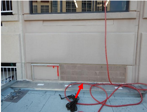
Figure 60. Roof-to-transition at the Green Garage. Metal expansion joint flashing sealed to precast panels and CMU infill (arrow).
