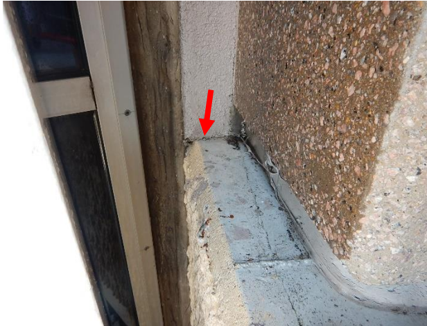
Figure 50. Vertical expansion joint between the skybridge and the Purple Garage. Water intrusion observed when spray testing the adjacent precast ledge after approximately 2 minutes.
