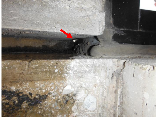
Figure 65. Daylight observed at corner of 2nd floor window sill above the roof-to-wall transition of the skybridge.
