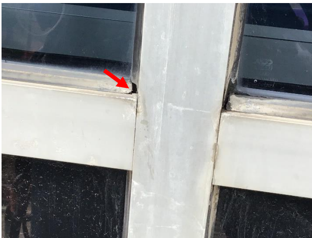
Figure 6. Gasket shrinkage at horizontal mullion.
