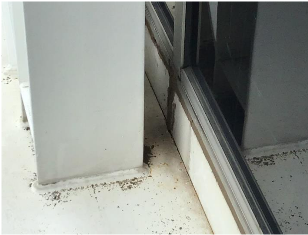
Figure 12. Butt joint in perimeter steel plate for the floor slab. Sealant inconsistently applied at joint.
