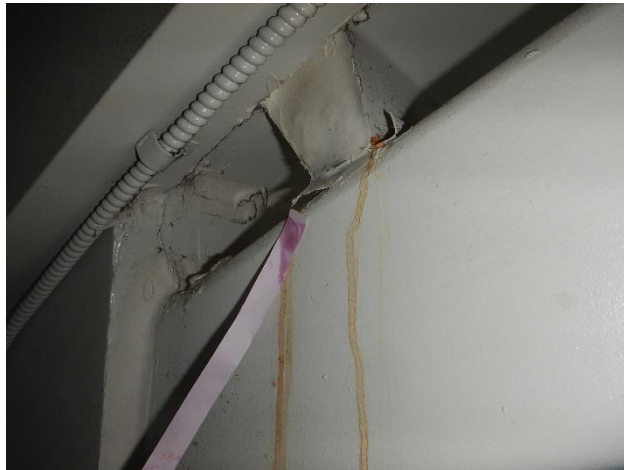
Figure 25. Water running out of metal deck flutes directly below sidewall transition.
