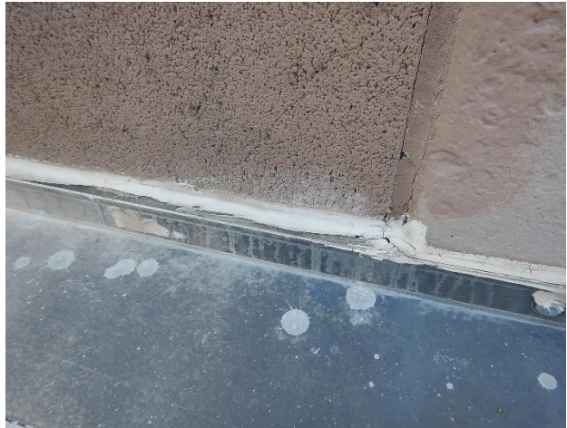
Figure 61. Deteriorated remedial sealant joint along top of expansion joint flashing.
