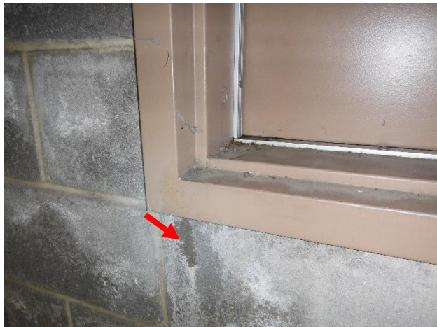
Figure 71. Water intrusion observed after 30 seconds of testing the metal access door.
