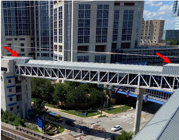
Figure 18. Low-slope roof areas at each end of the skybridge.
