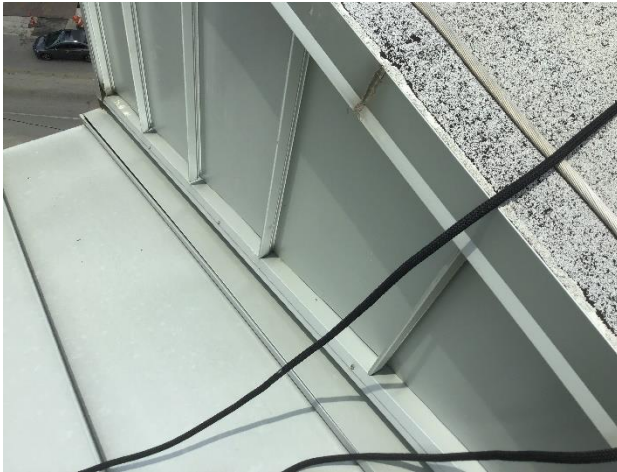
Figure 42. Sidewall transition at north end of Skybridge B.
