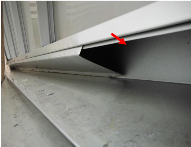
Figure 20. Section of missing counterflashing along sidewall roof transition.
