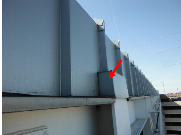
Figure 35. Sheet metal cap above steel column. Perimeter of cap not sealed at this location.
