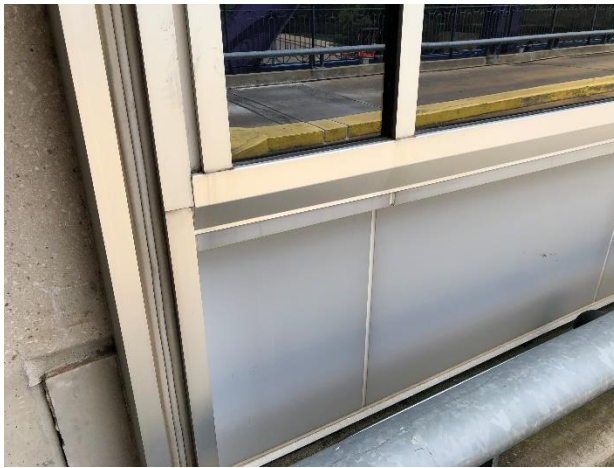
Figure 58. Vertical expansion joint at east end of Skybridge C. Photo also shows orientation of window system and metal panels below
