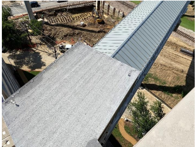
Figure 43. Low-slope roof at south end of Skybridge B.
