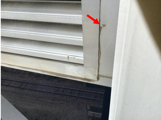
Figure 8. Louver set into window wall. Sealant around perimeter not consistently observed (arrow).
