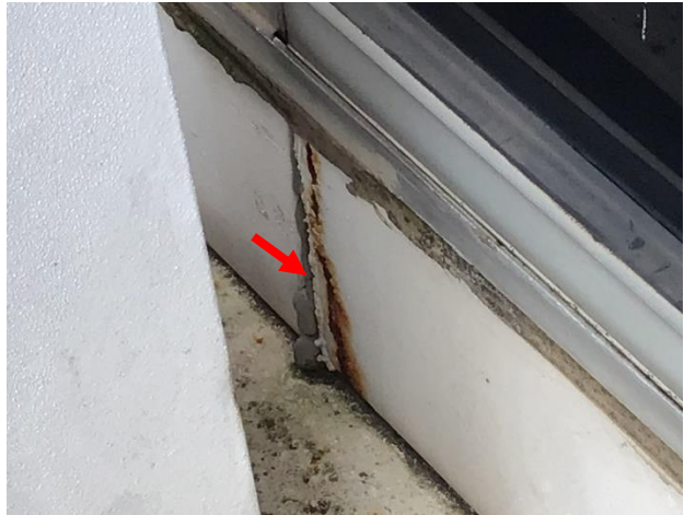
Figure 13. Corrosion at butt joint in the perimeter steel plate for the floor slab.
