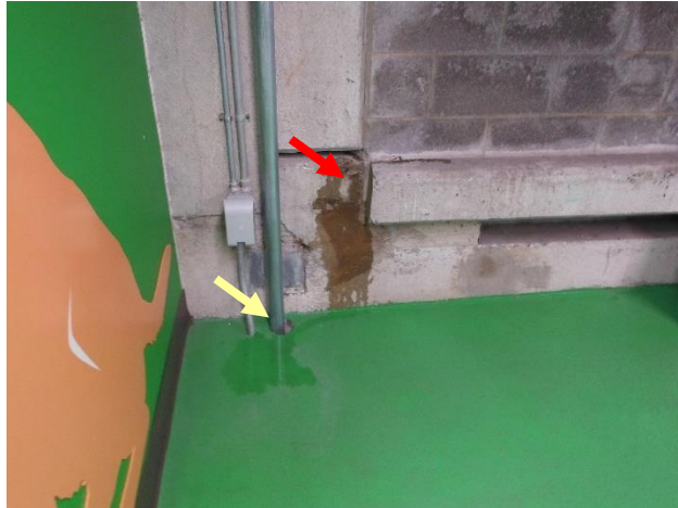
Figure 69. Water intrusion (red arrow) observed when spraying cracks/separations within the CMU infill above the roof-to-wall transition. Water migrated down through conduit penetrations within the garage floor (yellow arrow).
