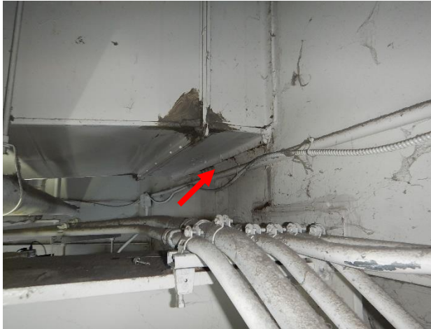
Figure 30. Water staining observed below intersection of duct work and exterior wall behind louver within the metal wall panels on the west facade.
