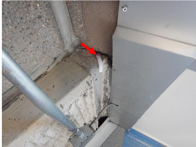
Figure 51. Water intrusion observed on top of precast ledge.
