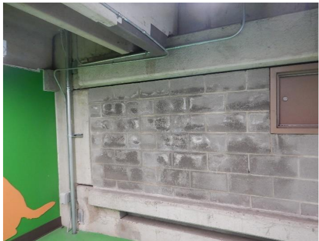
Figure 63. Efflorescence and water staining on back of CMU infill.
