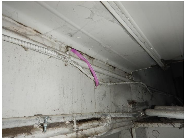
Figure 49. Water intrusion observed running out of the bottom joint between the louver duct work and the wall.
