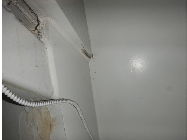
Figure 23. Water intrusion running out from behind drywall at south exterior wall when testing sidewall transition above.
