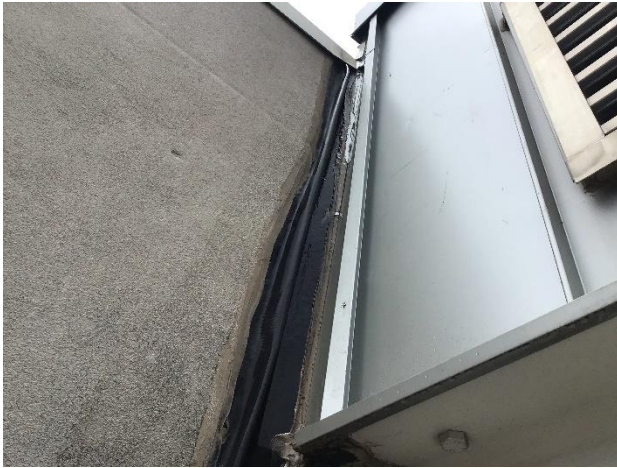
Figure 16. Black flexible membrane at west termination of skybridge. Edges of membrane sealed with sealant.
