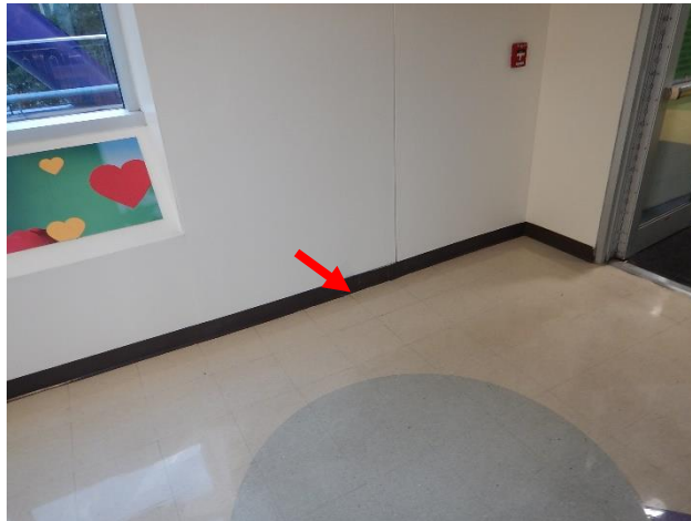
Figure 75. Water intrusion observed at base of wall behind windows.
