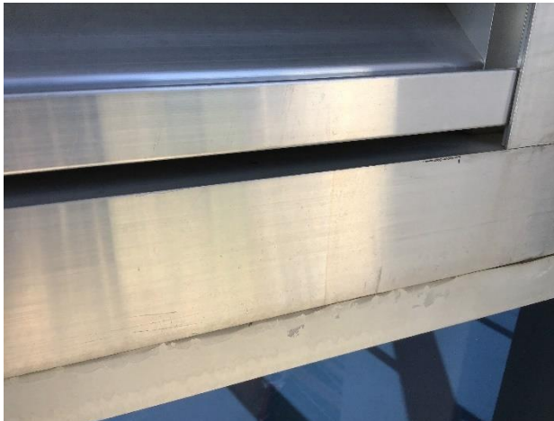
Figure 32. Base of louver within window wall.
