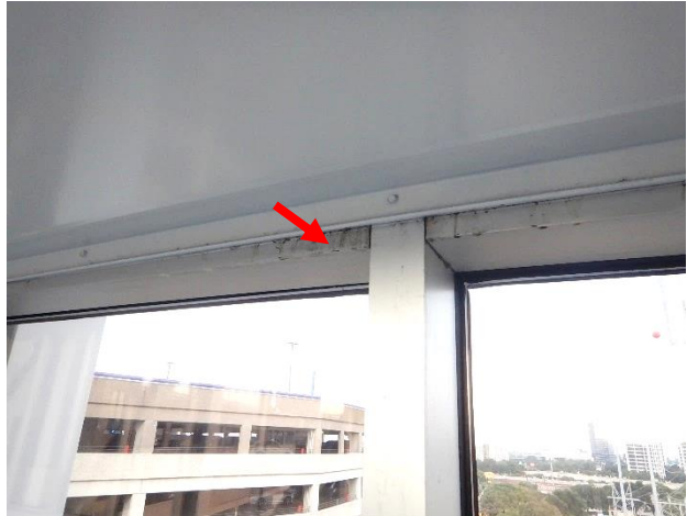
Figure 31. Water stains below louvers within window wall.
