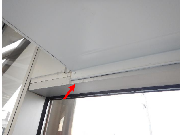
Figure 5. Water stains below louvers within window wall.
