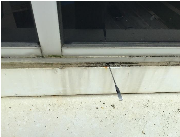
Figure 10. Dirt build-up and organic growth around weep in perimeter sealant joint at sill and along top edge of sill receiver. Photo shows probe inserted into weep hole within sill receiver.
