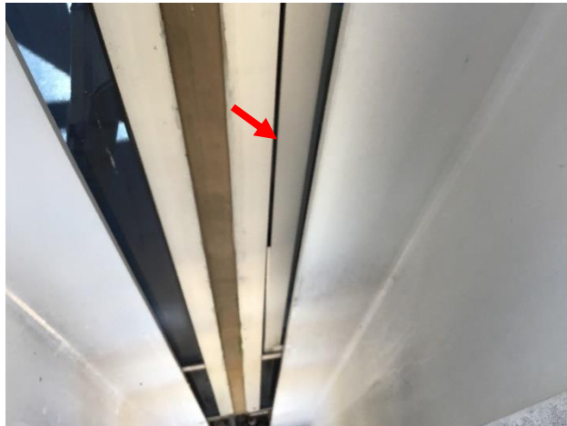
Figure 37. Unsealed joint between window wall frame and inset operable window frame.
