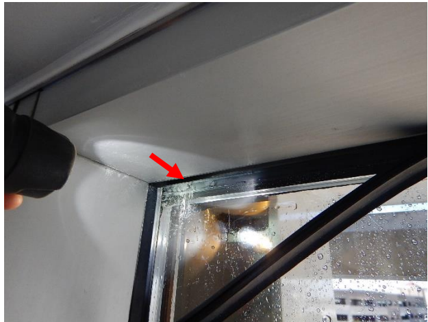
Figure 29. Removal of interior head gasket revealed that the top of the glass was in line with the daylight opening of the frame.
