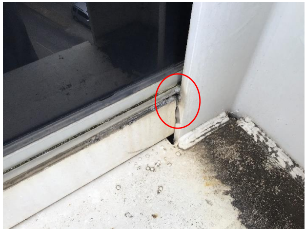
Figure 11. Dirt build-up and organic growth around weep in perimeter sealant joint at sill and along top edge of sill receiver. Photo shows probe inserted into weep behind steel column. Condition of sealant joint behind column could not be observed.
