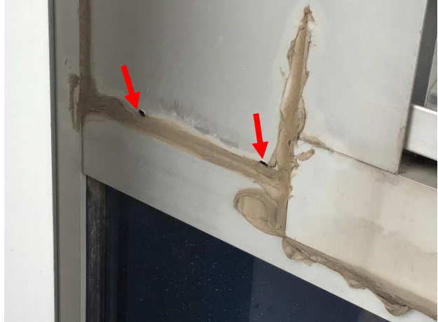
Figure 9. Weep holes observed at bottom on infill panel adjacent to east louver on the south facade.
