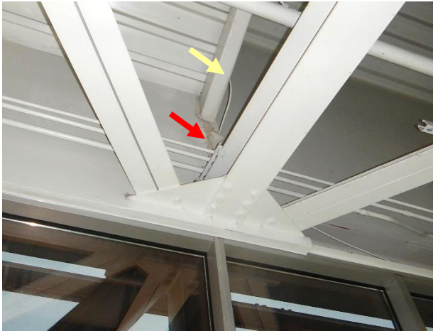
Figure 4. Water stains on steel framing (yellow arrow) and peeling paint on drywall (red arrow) below sidewall roof transition.
