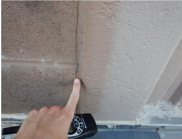
Figure 68. Separation/cracks were tested within the CMU infill above the roof-to-wall transition.
