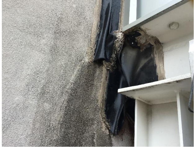
Figure 17. Black flexible membrane at west termination of skybridge. Edges of membrane sealed with sealant.
