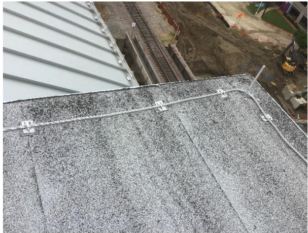
Figure 19. Typical granule loss observed at the roof membrane at the low-slope roof areas.
