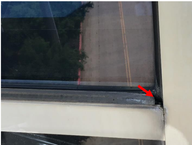
Figure 36. Gasket shrinkage on east facade.
