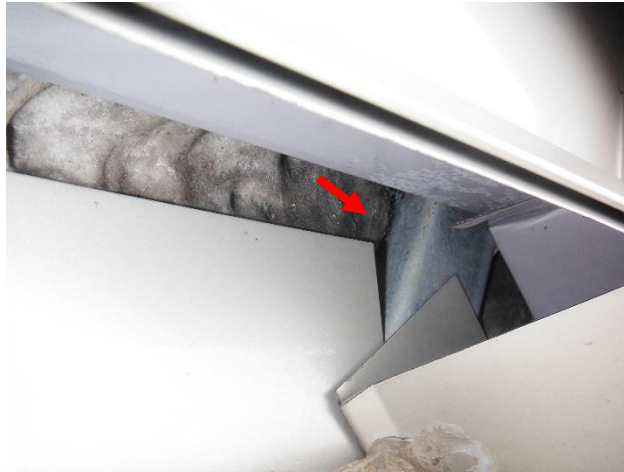
Figure 21. Insulation and framing observed behind section of missing counterflashing.
