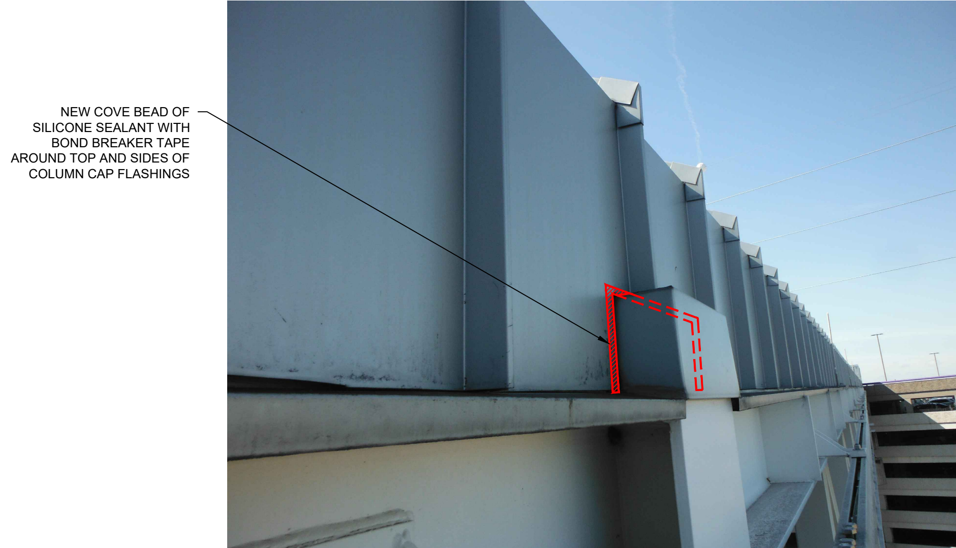
C6 Sealant Joint at Column Cap Flashing SCALE: 3" = 1'-0"
