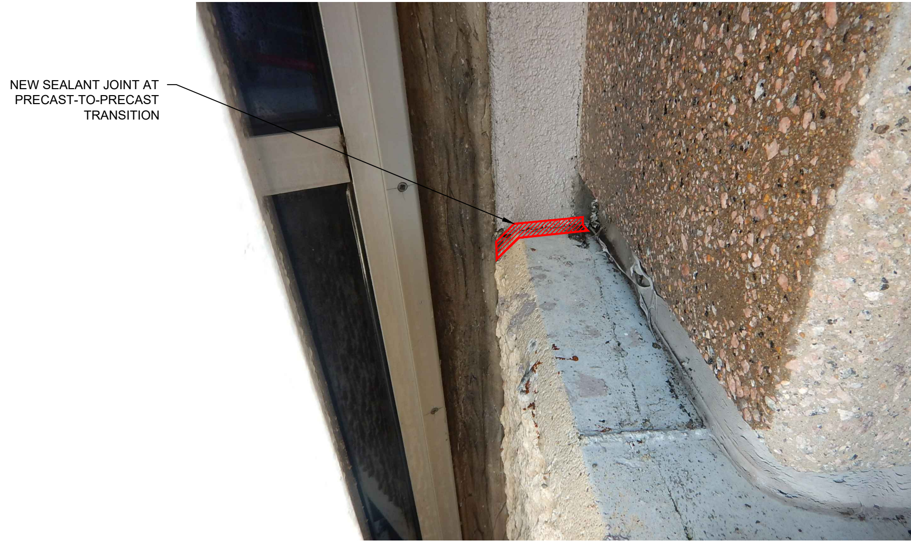
A6 Sealant Repair at Precast to Precast Joint SCALE: 3" = 1'-0"
