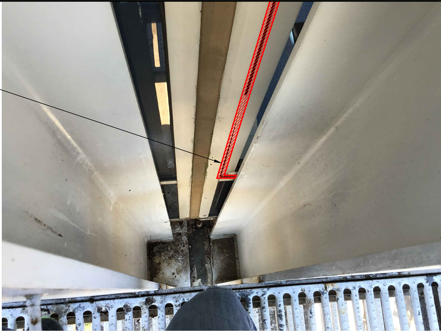
E6 Sealant Repair at Open Window Joint SCALE: 3" = 1'-0"
