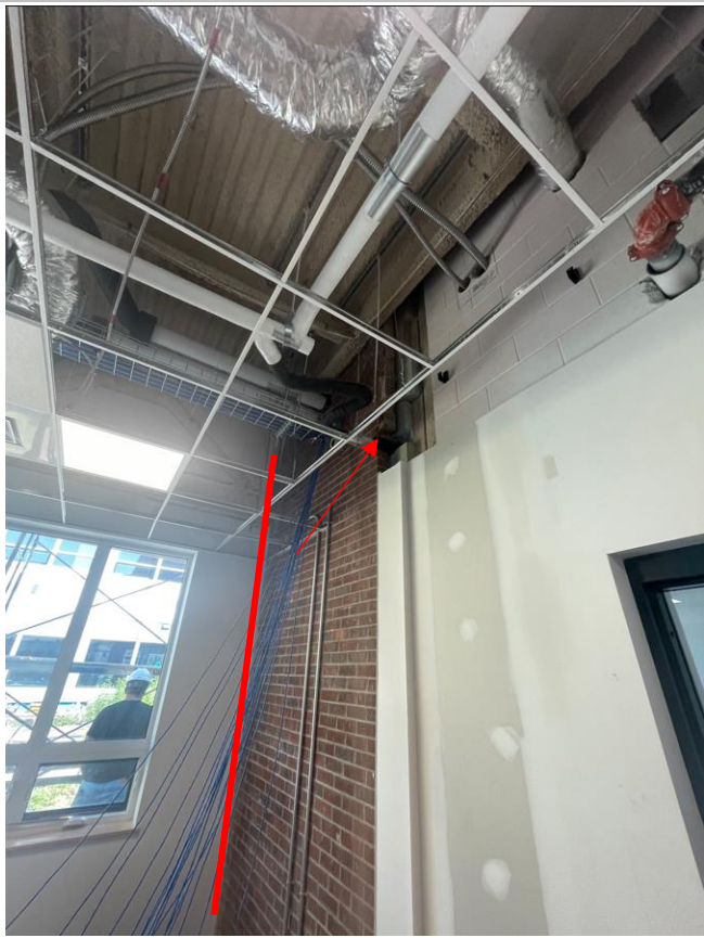
The tested transition is outlined above. Pointed to above is an air bypass through the existing layers which is described in the next table.
