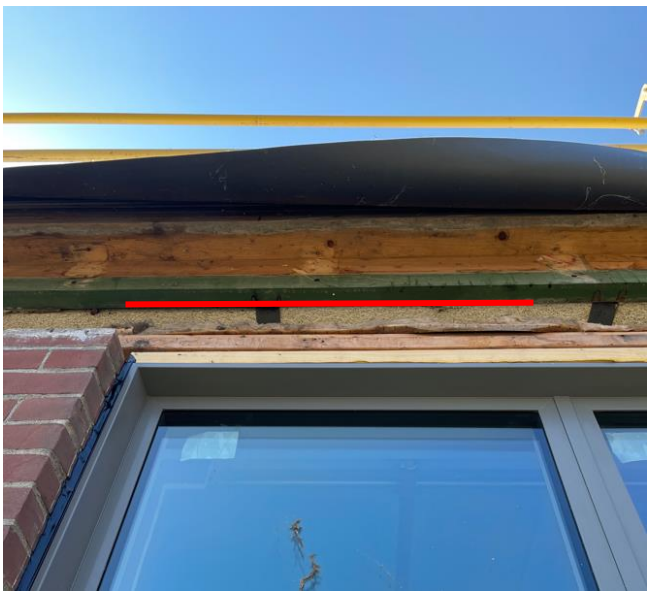
Close up image showing another location where fog was observed to escape during testing.
