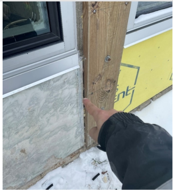
Break in the air seal along the granite transition. This transition leaked heavily.
