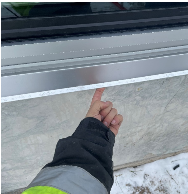
Fog leaked heavily underneath the sill flashing. The sill flashing is sealed to the wood buck; however, the wood buck does not appear to be sealed to the exterior granite.
