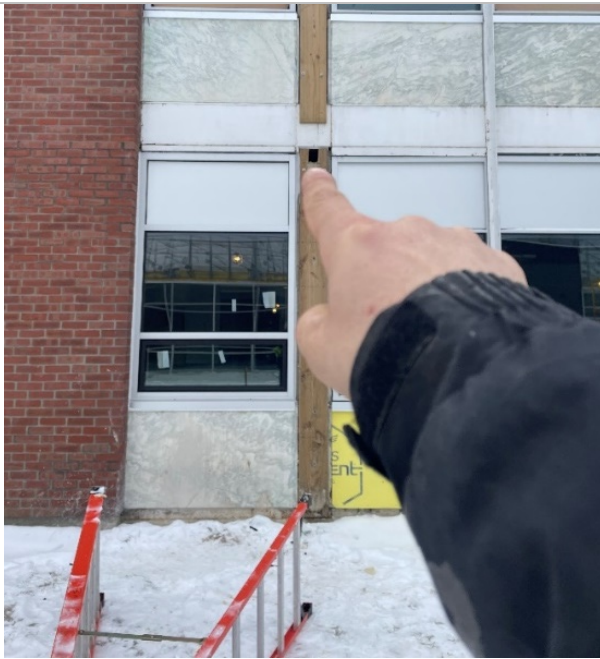
Hole in wood covering over concrete column. What is the plan for addressing this - can foam?
