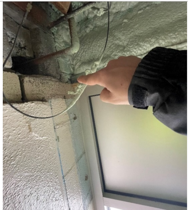
Heavy leakage at top corners of the curtain wall. From the right angle, daylight is visible through this. Caulk can be added from inside to the area pointed at above. Same leakage occurred at the opposite side of the head as well.
