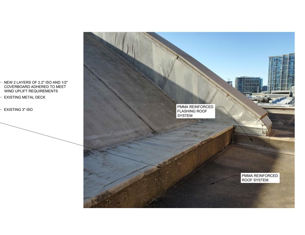
ROOF RAKE STONE COPING DETAIL ON DOME
