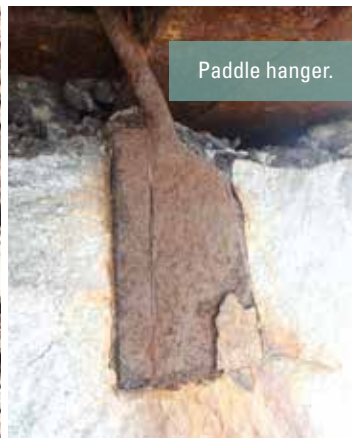
Typical steel assembly, note gap is at location of failed stone.
