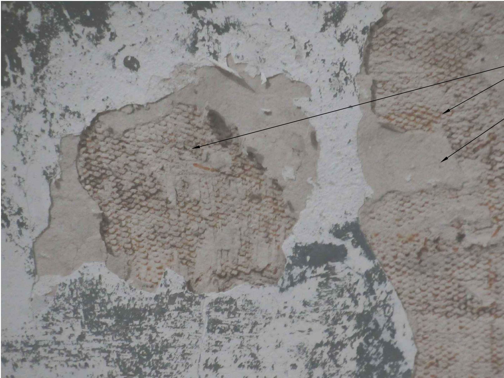
A5 Enlarged View of Plaster Delaminations SCALE: 1 1/2" = 1'-0"
