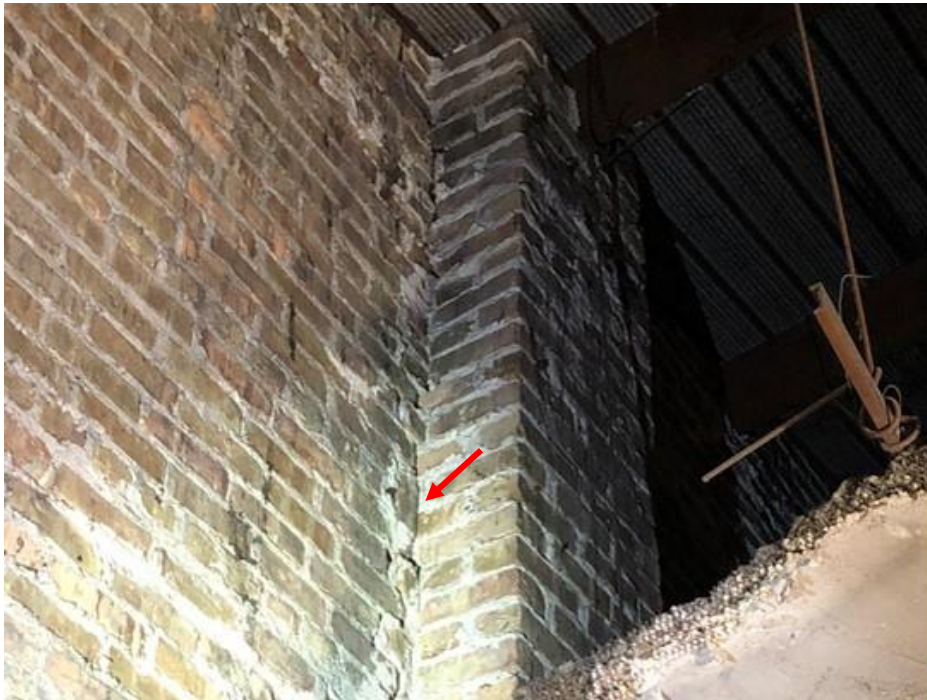
Figure 5. View of gap at pier to wall interface at south pier (arrow)
