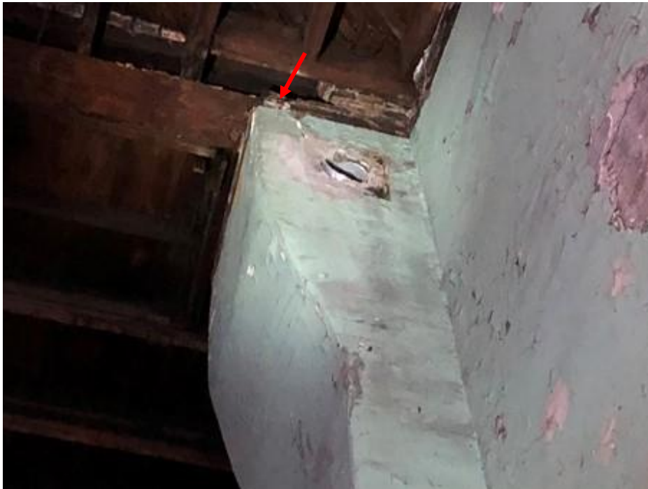
Figure 8. View of steel beam bearing on corbeled masonry chimney (arrow)
