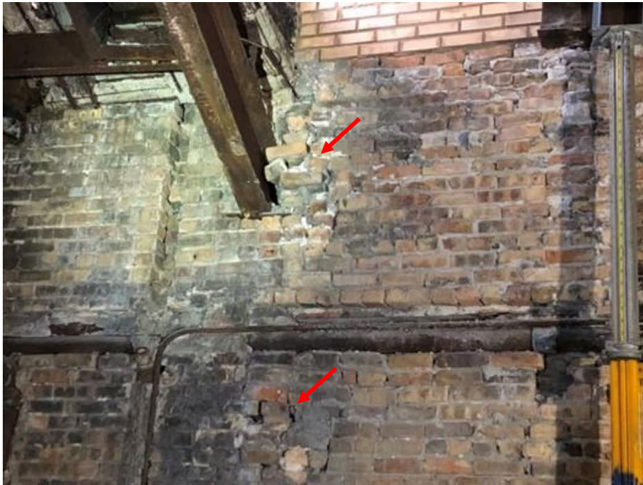
Figure 1. View of distressed masonry adjacent to embedded steel (arrows)
