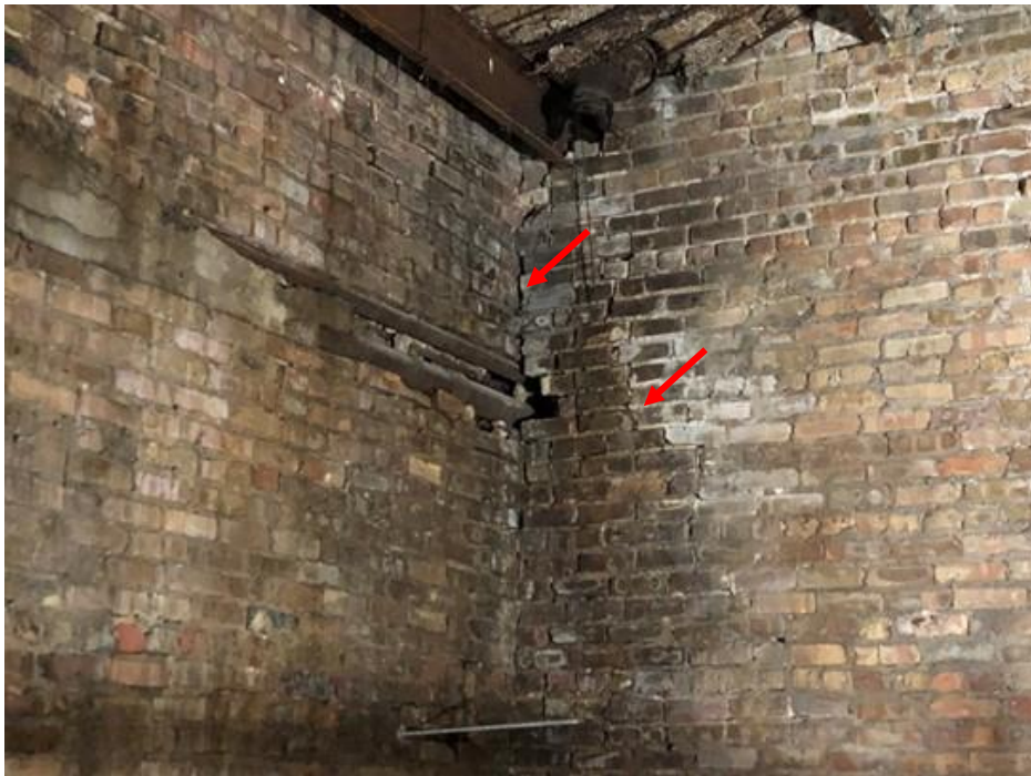
Figure 2. View of cracking at southwest corner (arrows)
