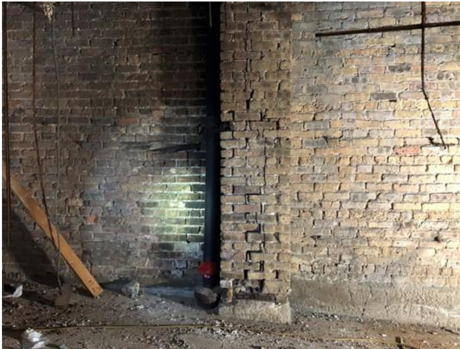
Figure 3. View of distress at the lower 5 feet of the center pier
