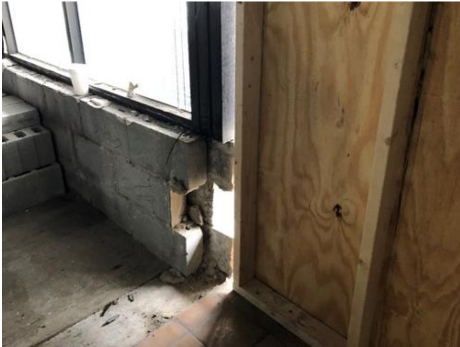
Figure 9. View of opening for new limestone knee wall
