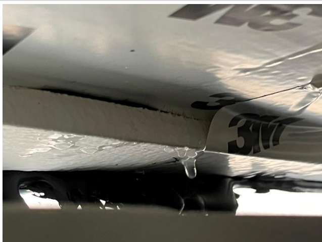
Photo 16 – View of moisture intrusion observed at interior.
