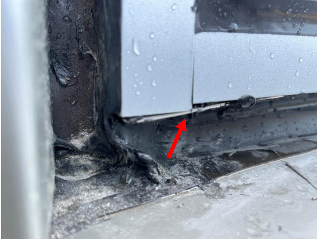
Photo 25 – Enlarged exterior view of moisture intrusion location.
