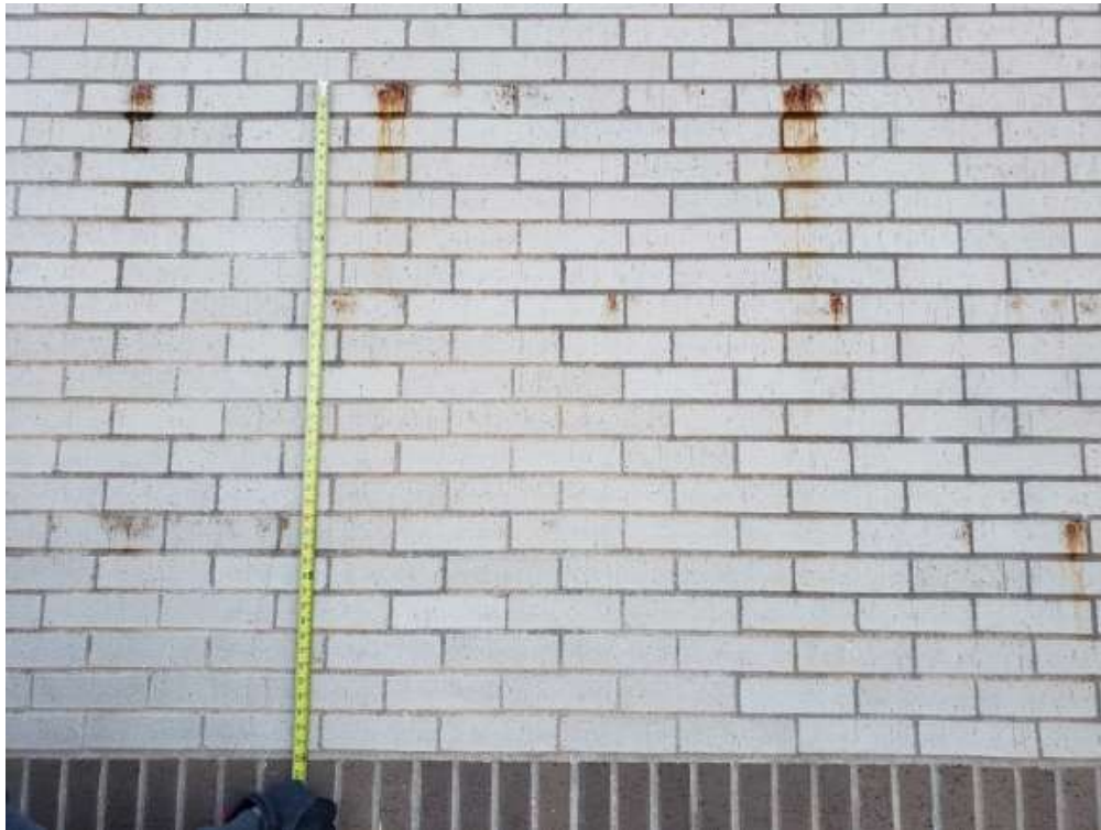
Photo #108: Representative example of predominate rust stains at vertical intervals of approximately 16" on-center, which was 6 mortar bed joints (north elevation, stairwell, 1/12/22).
