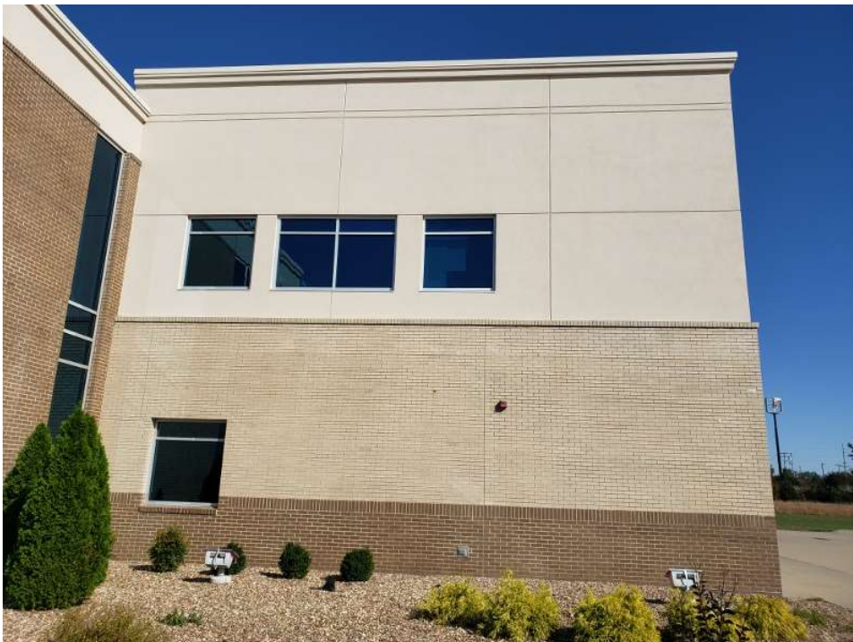
Photo #75: View of orange/red staining and white residue on the brick (west elevation, south of lobby, 10/18/21).
