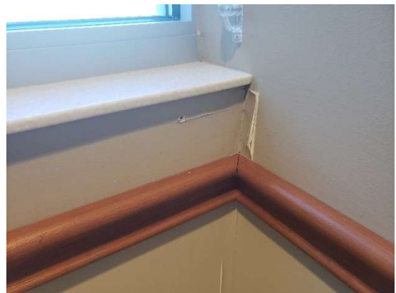
Photo #18: Chipped paint on drywall at the bottom of the window jamb rough opening at leak location #10.
