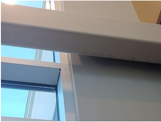
Photo #7: Drip marks on the bottom side of the horizontal steel tubing at leak location #3.
