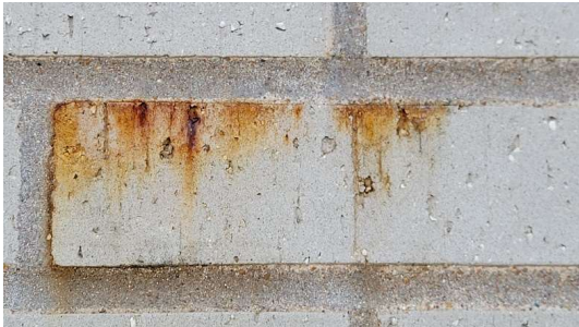
Photo #86: Close-up view of orange/red staining on the brick (west elevation, gymnasium, 1/11/22).
