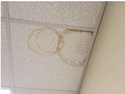
Photo #29: Stains on the ceiling tile at leak location #20.
