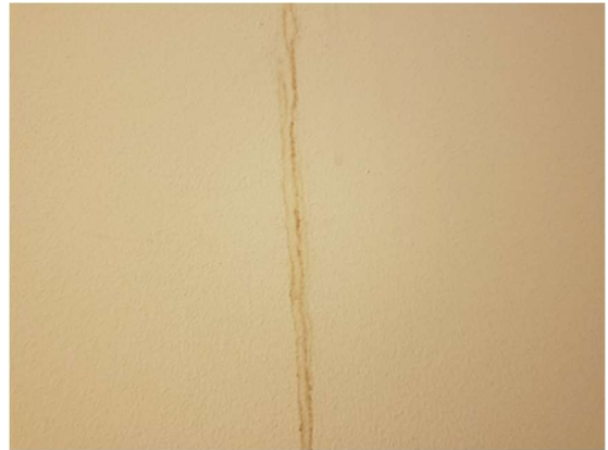
Photo #14: Stains on drywall at leak location #8.
