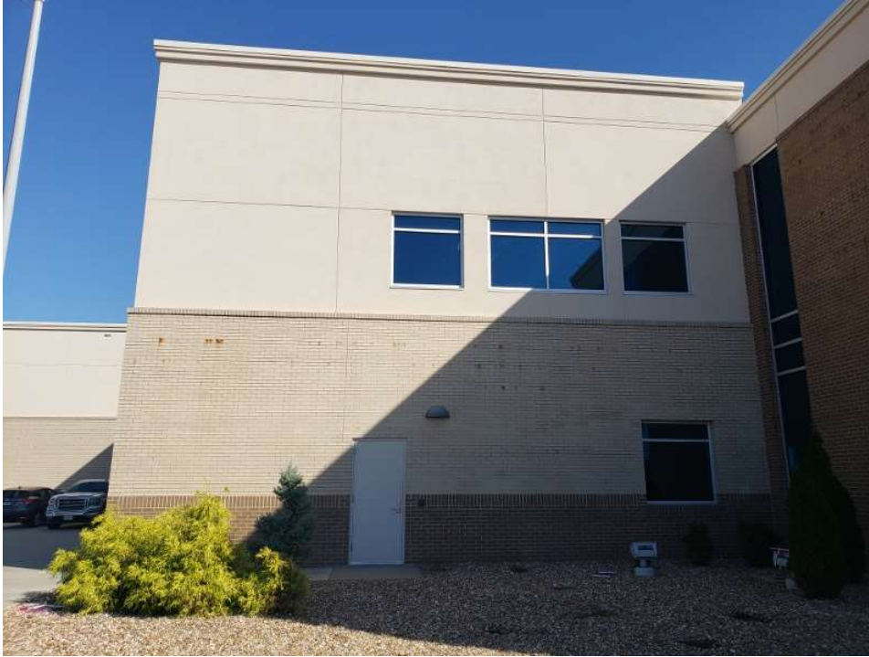
Photo #74: View of orange/red staining and white residue on the brick (west elevation, north of lobby, 10/18/21).
