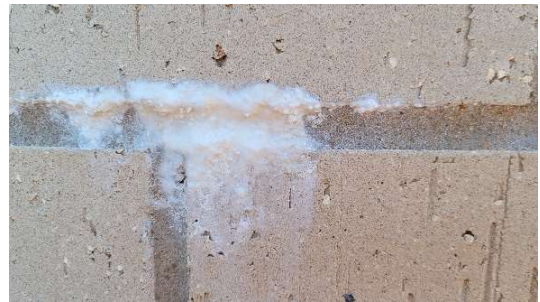
Photo #90: Close-up view of white residue on the brick (west elevation, gymnasium, 1/11/22).
