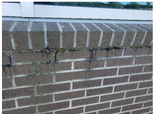
Photo #96: Close-up view of white residue on the brick (north elevation, fitness area, 10/18/21).
