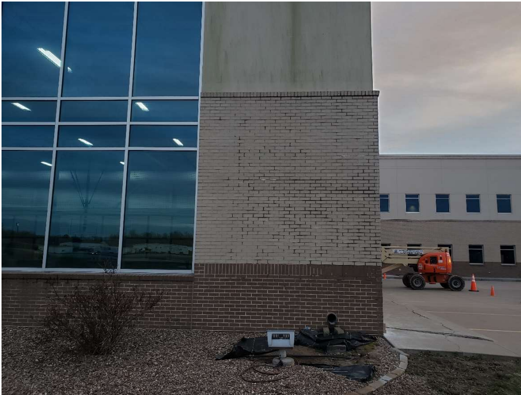
Photo #80: View of dark residue on the mortar (north elevation, gymnasium, 1/12/22).
