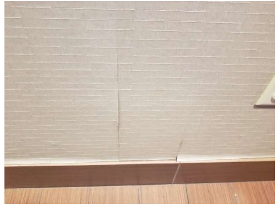
Photo #8: Wallpaper peeling below the window at leak location #5.
