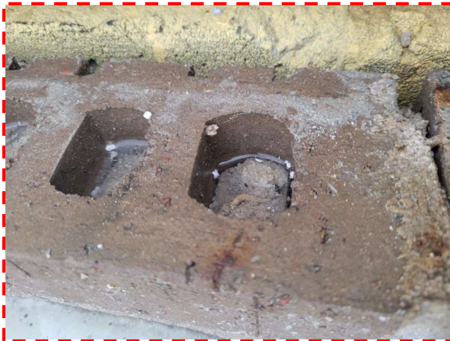
Photo #115: Close-up view of water in brick cores at the base-of-wall condition (north elevation, stairwell, 7/19/23).
