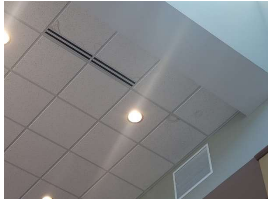
Photo #26: Stains on the ceiling tiles at leak location #17.
