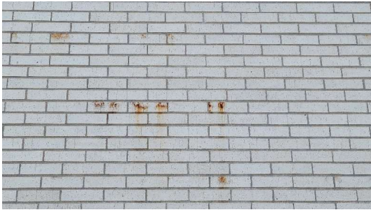
Photo #84: Close-up view of orange/red staining on the brick (west elevation, gymnasium, 1/11/22).
