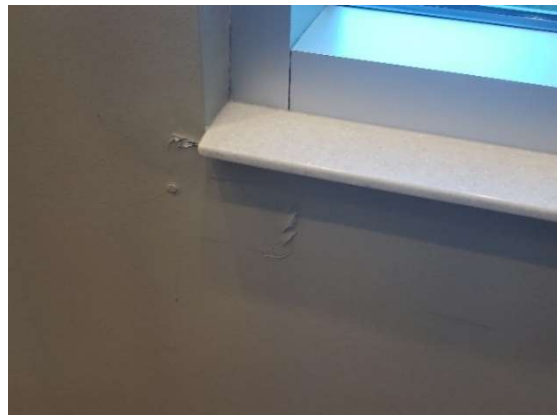
Photo #6: Chipped paint on drywall at the bottom of the window jamb rough opening at leak location #3.
