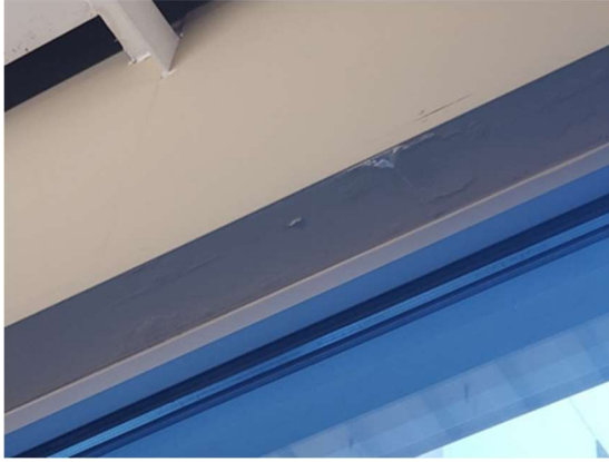
Photo #1: Chipped paint on drywall along the top of the window rough opening at leak location #1.
