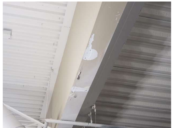
Photo #22: Chipped paint on drywall along the spandrel beam at leak location #13.
