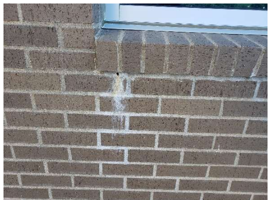
Photo #97: Close-up view of white residue on the brick (north elevation, fitness area, 10/18/21).
