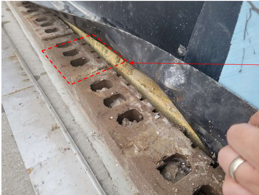
Photo #114: View underneath unsealed flashing membrane at the base-of-wall condition (north elevation, stairwell, 7/19/23).
