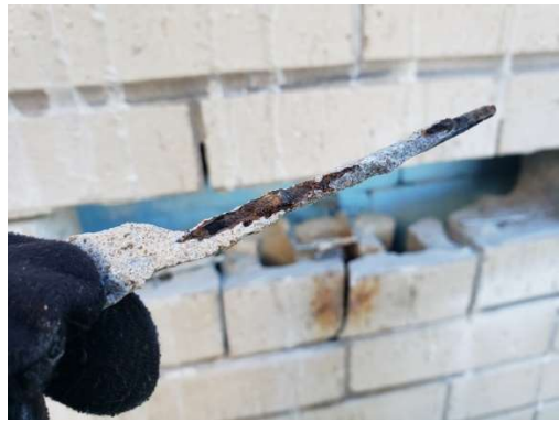
Photo #103: Close-up view of corroded brick wire (north elevation, fitness area, 1/10/22)
