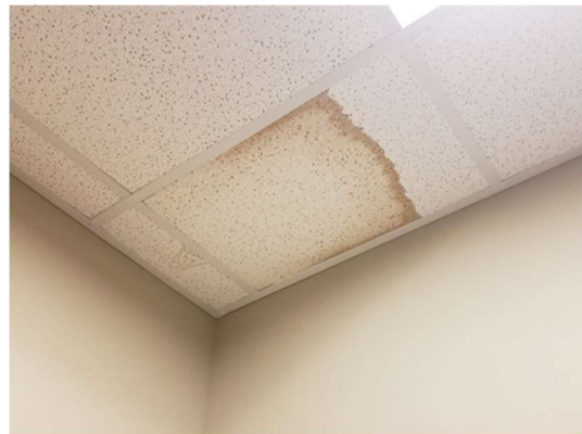
Photo #30: Stains on the ceiling tiles at leak location #21.
