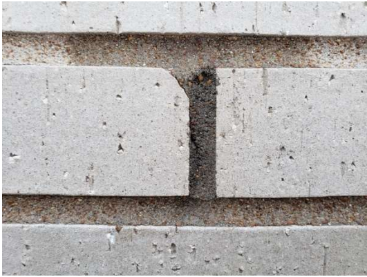
Photo #92: Close-up view of wet mortar (north elevation, gymnasium, 1/12/22).
