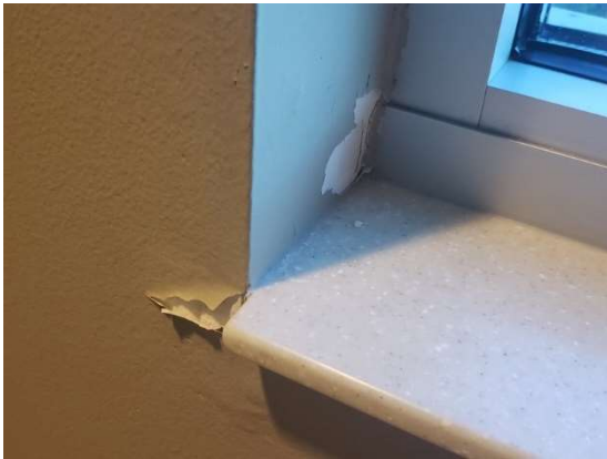
Photo #3: Chipped paint on drywall at the bottom of the window jamb rough opening at leak location #2.
