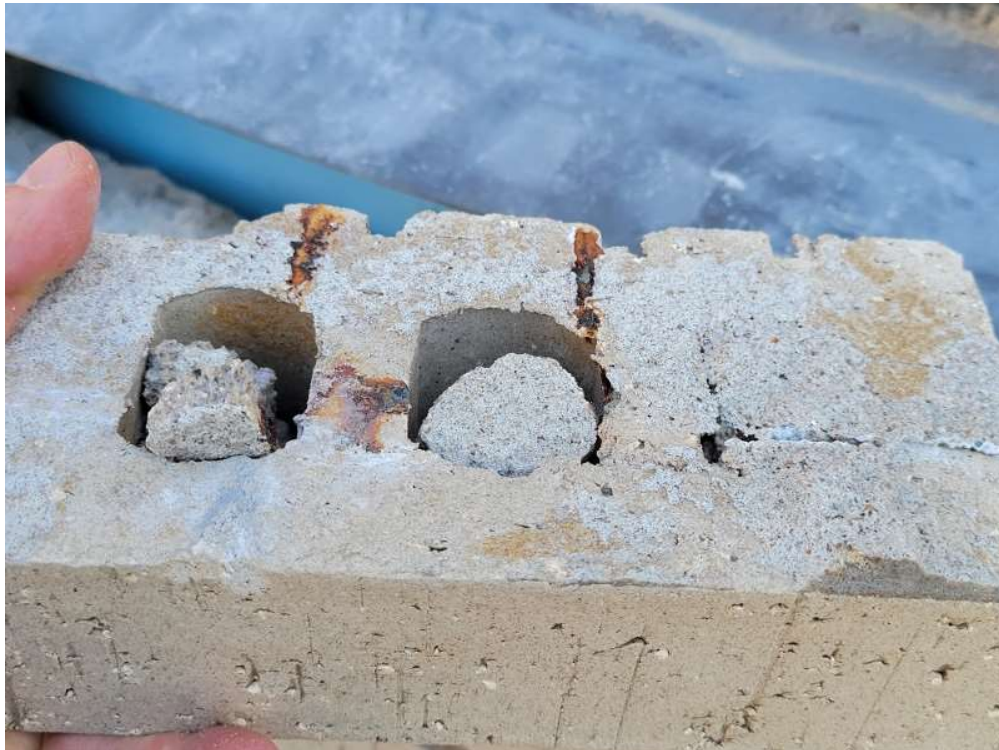
Photo #118: Rust stains on the top side of a brick unit after removal of the brick anchor tie (north elevation, fitness area, 6/26/23).
