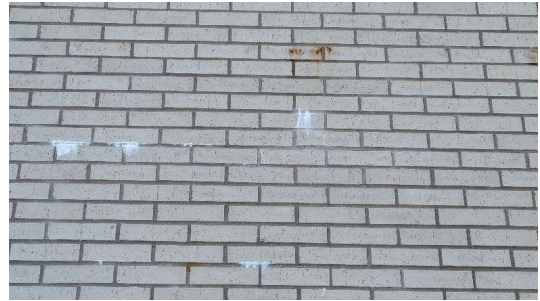
Photo #85: Close-up view of orange/red staining and white residue on the brick (west elevation, gymnasium, 1/11/22).
