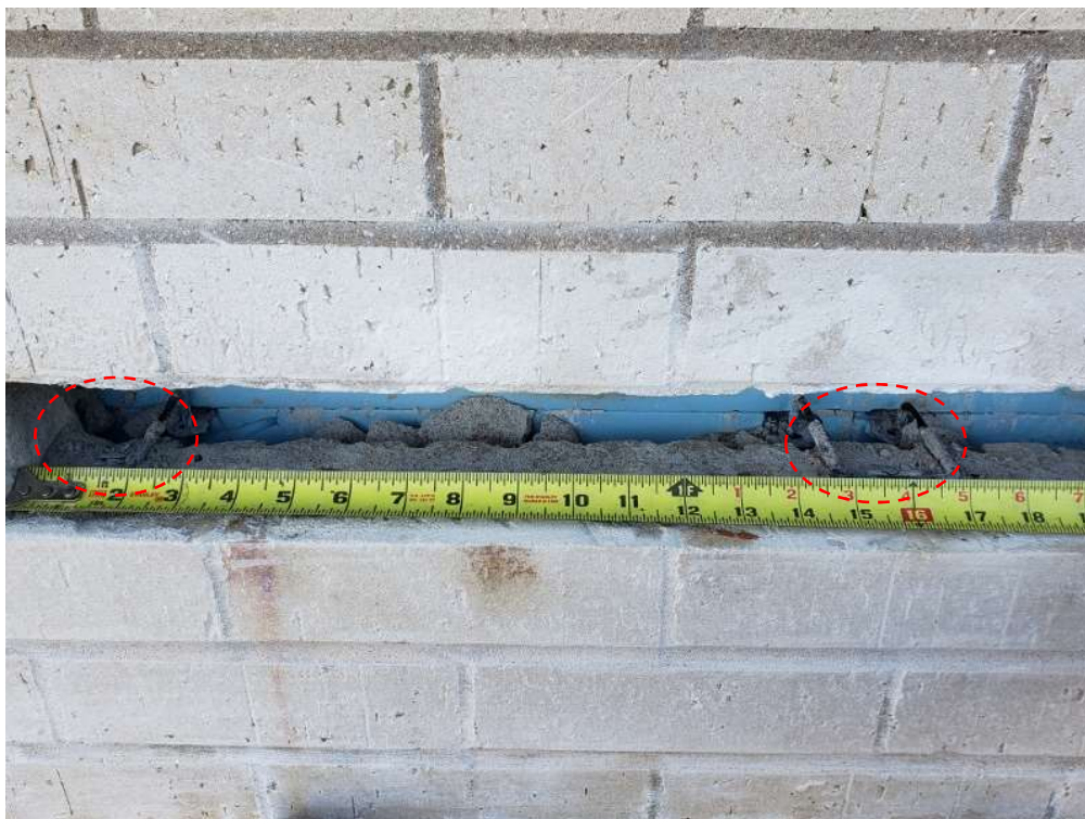
Photo #107: Representative example of brick anchor tie horizontal spacing of approximately 16" on-center (west elevation, stairwell, 1/12/22).
