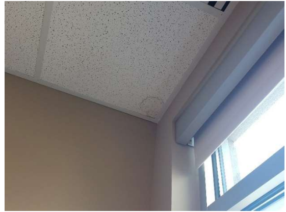
Photo #20: Stain on the ceiling tile directly above the window at leak location #11.
