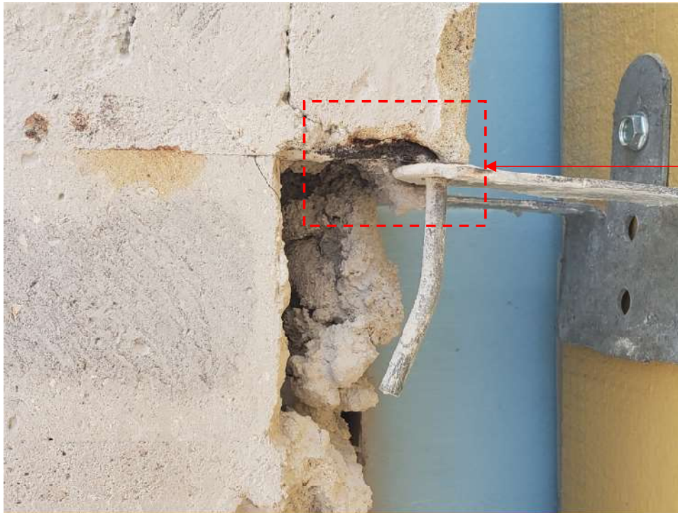
Photo #128: View of a rusted brick wire, but no indication of steel corrosion where not embedded in the mortar joint (west elevation, stairwell, 8/30/23).
