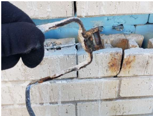
Photo #102: Close-up view of corroded brick anchor tie (north elevation, fitness area, 1/10/22).
