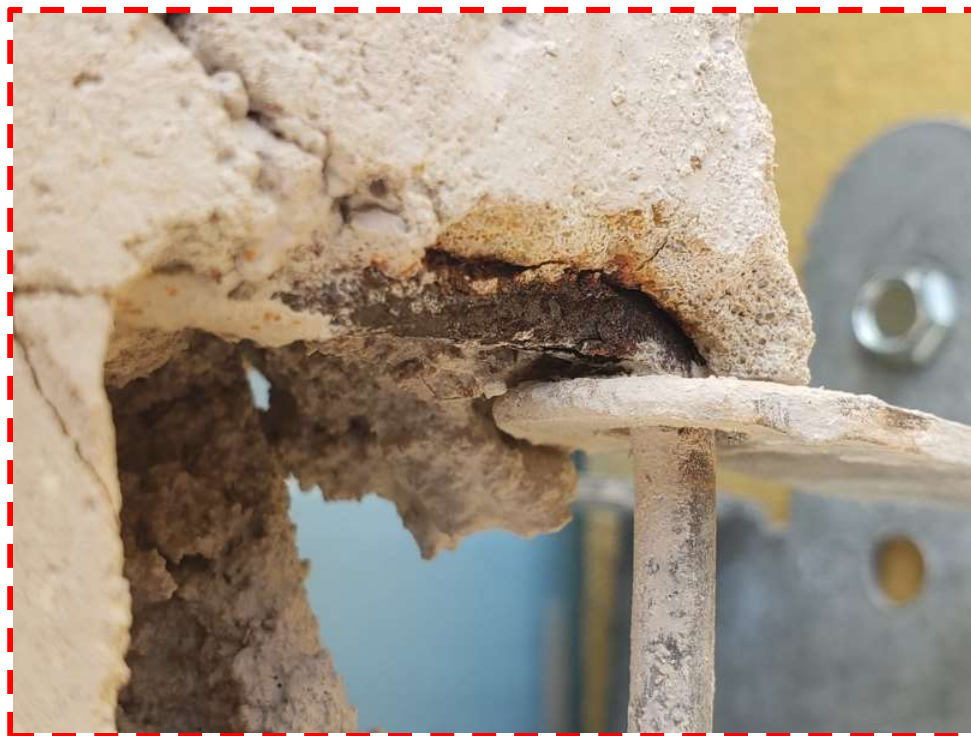
Photo #129: Close-up view of rusted brick tie in direct contact with the mortar, but no indication of steel corrosion where not embedded in the mortar joint (west elevation, stairwell, 8/30/23).
