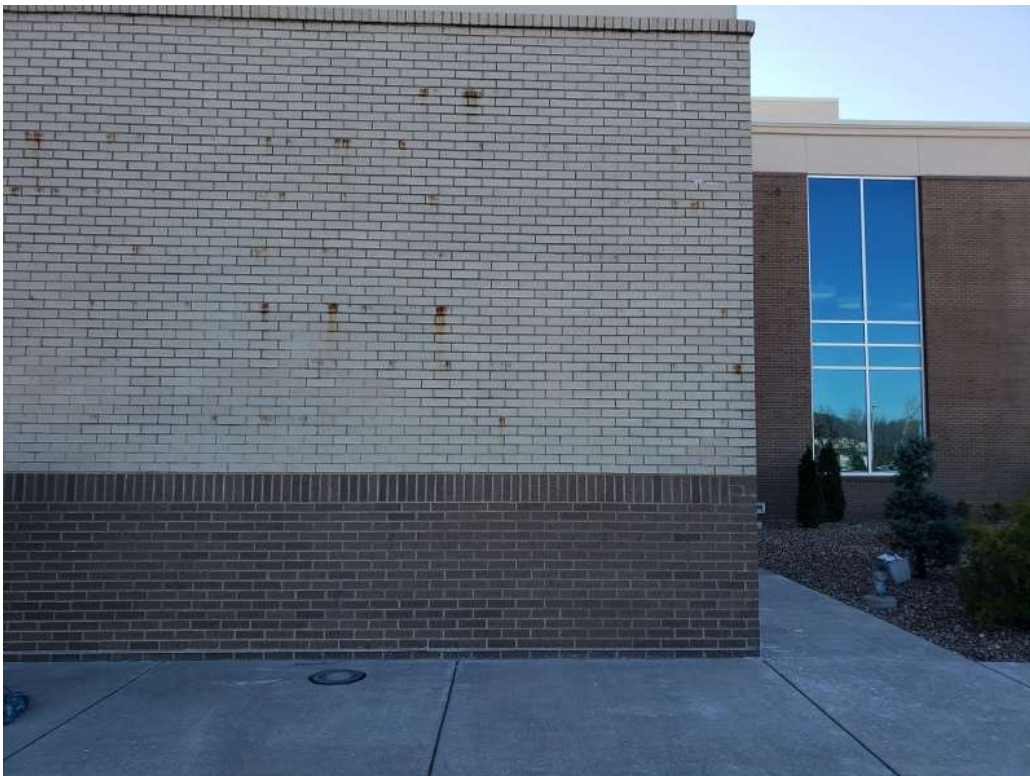
Photo #77: View of orange/red staining and white residue on the brick (north elevation, stairwell, 1/12/22).
