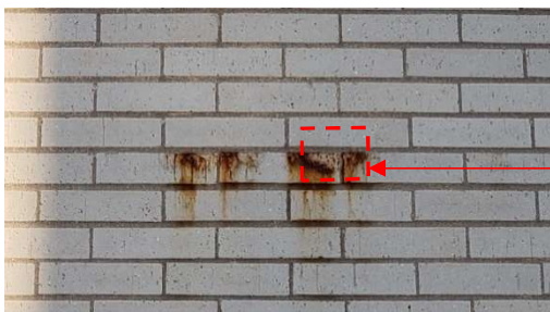
Photo #104: View of rust stain on brick surface, prior to exploratory opening (west elevation, stairwell, 1/10/22).
