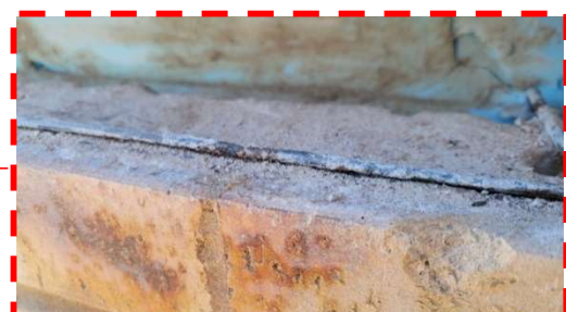
Photo #105: Close-up view of corroded brick wire (west elevation, stairwell, 1/10/22).
