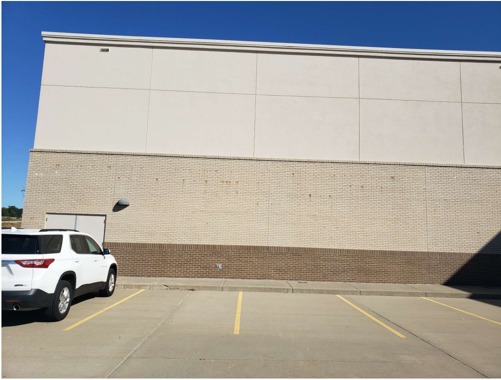
Photo #76: View of orange/red staining and white residue on the brick (west elevation, gymnasium, 10/18/21).
