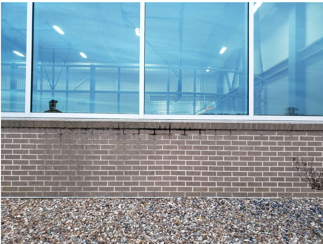
Photo #81: View of dark residue on the mortar (north elevation, gymnasium, 10/18/21).
