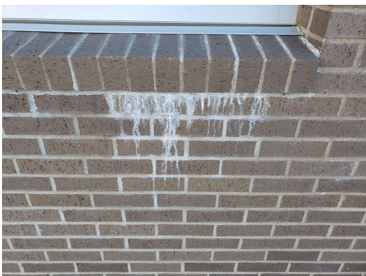
Photo #94: Close-up view of white residue on the brick (north elevation, fitness area, 10/18/21).
