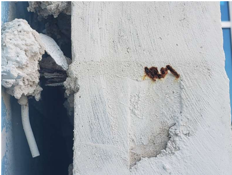
Photo #125: View of a rusted brick anchor tie and wire, but no indication of staining on the brick surface (west elevation, hallway, 8/30/23).
