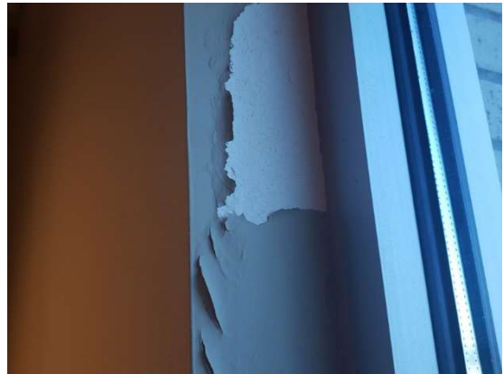
Photo #4: Chipped paint on drywall along the window jamb rough opening at leak location #2.
