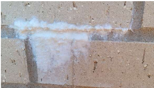
Photo #87: Close-up view of white residue on the brick (west elevation, gymnasium, 1/11/22).
