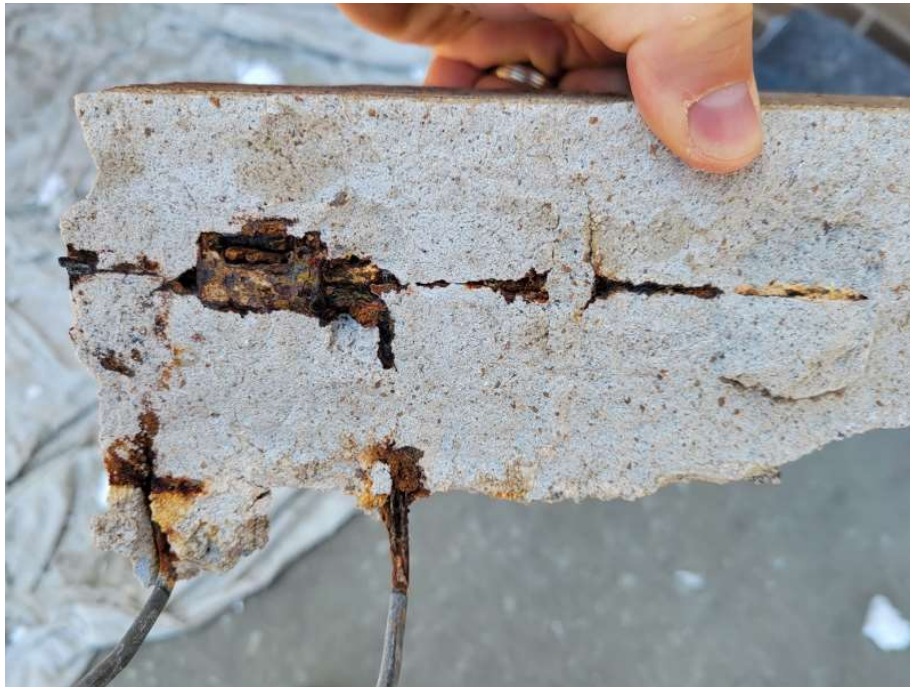
Photo #116: Underside view of a brick unit with a corroded brick anchor tie and wire, embedded in the mortar (north elevation, fitness area, 6/26/23).
