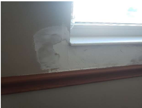
Photo #21: Presumable drywall repair at the bottom of the window jamb rough opening at leak location #12.
