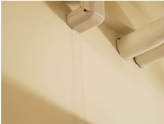
Photo #13: Stains on drywall at leak location #7.
