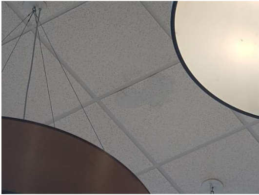
Photo #25: Stains on the ceiling tiles at leak location #16.
