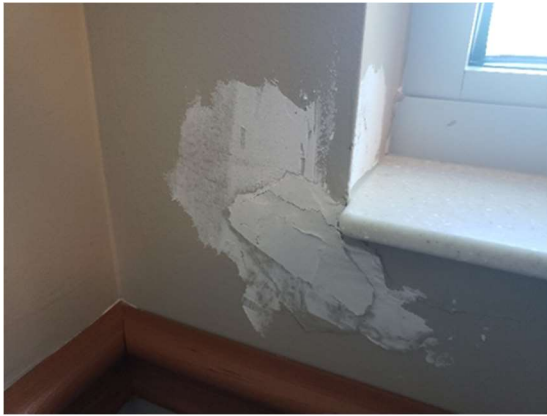
Photo #19: Presumable drywall repair at the bottom of the window jamb rough opening at leak location #11.
