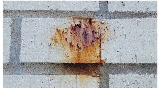
Photo #89: Close-up view of orange/red staining on the brick (west elevation, gymnasium, 1/11/22).
