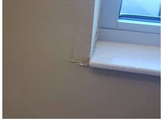
Photo #2: Chipped paint on drywall at the bottom of the window jamb rough opening at leak location #1.
