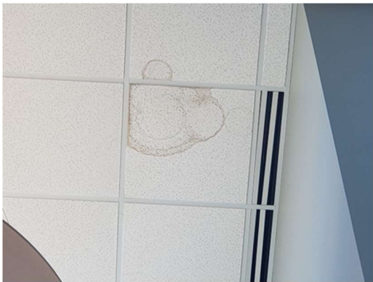
Photo #27: Stains on the ceiling tiles at leak location #18.
