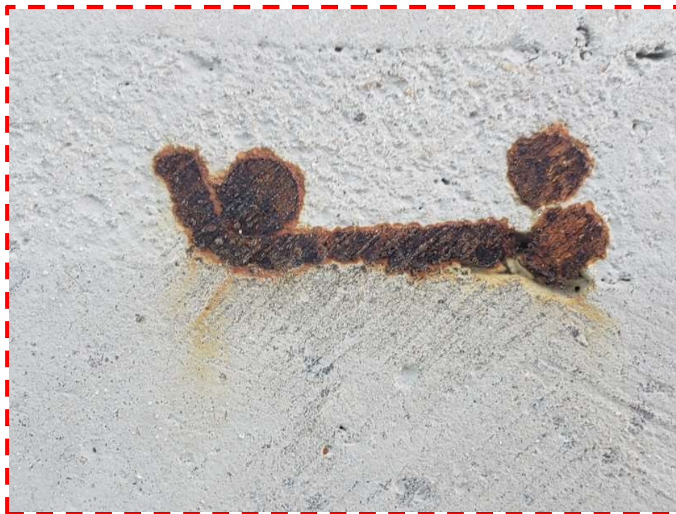
Photo #123: Close-up view of a rusted brick anchor tie and wire (west elevation, hallway, 8/30/23).
