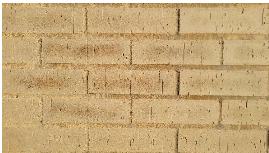
Photo #88: Close-up view of brick discoloration (south elevation, stairwell, 1/12/22).
