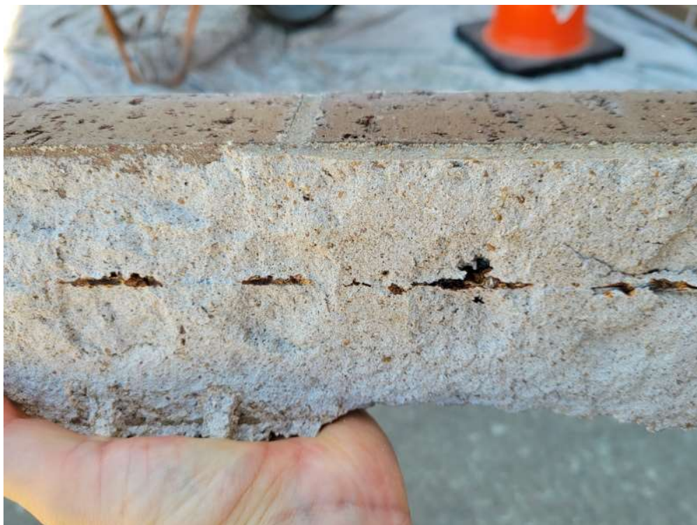
Photo #119: Rust stains on the mortar along a wire (north elevation, fitness area, 6/26/23).
