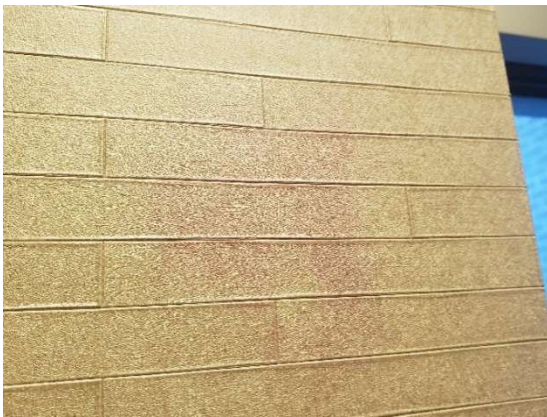
Photo #9: Wallpaper discoloration adjacent to the window at leak location #5.
