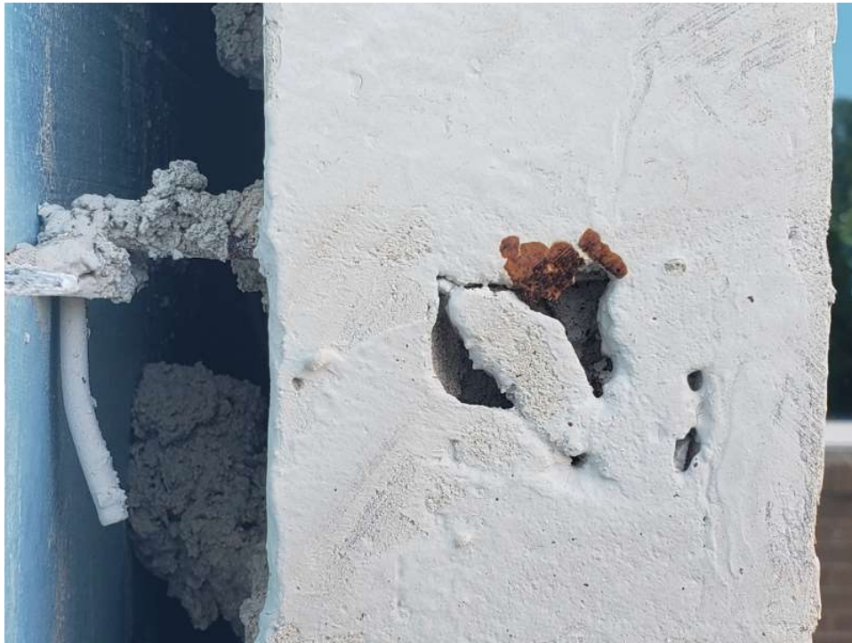
Photo #124: View of a rusted brick anchor tie and wire, but no indication of staining on the brick surface (west elevation, hallway, 8/30/23).
