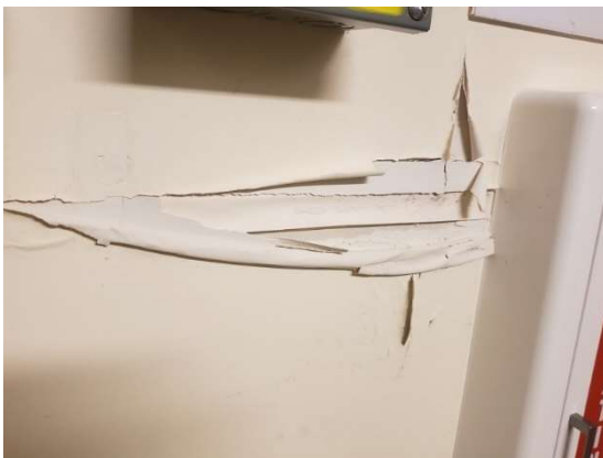
Photo #11: Chipped/peeling paint on drywall at leak location #6.
