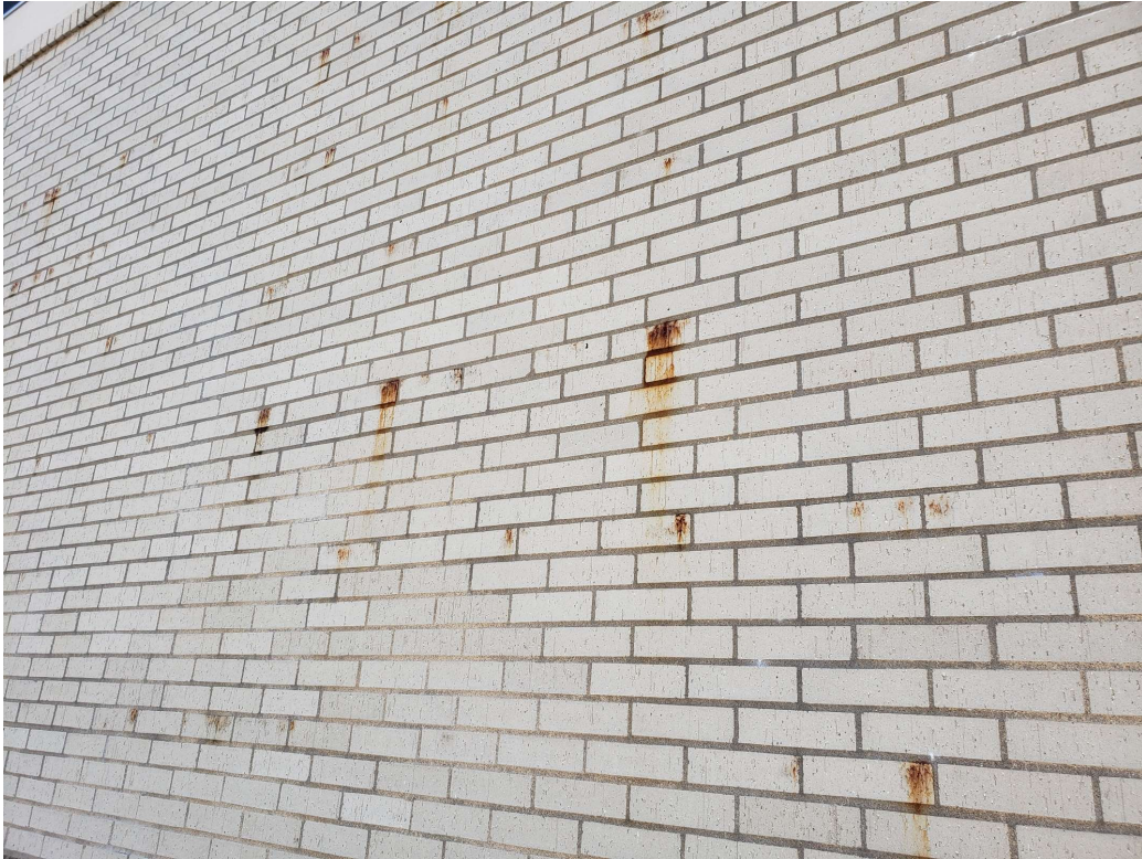
Photo #82: Close-up view of orange/red staining on the brick (north elevation, stairwell, 10/18/21).
