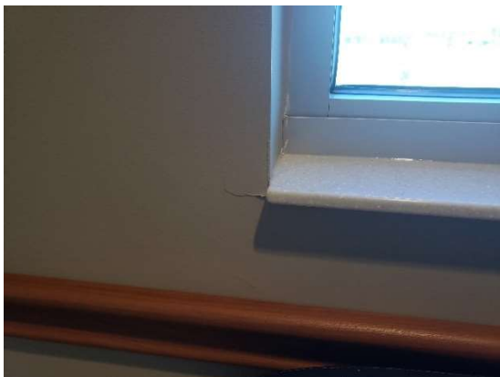
Photo #17: Chipped paint on drywall at the bottom of the window jamb rough opening at leak location #10.
