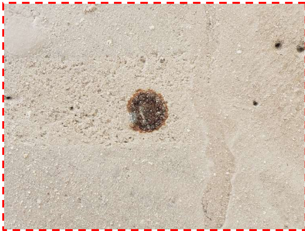
Photo #127: Close-up view of rusted brick wire (west elevation, stairwell, 8/30/23).
