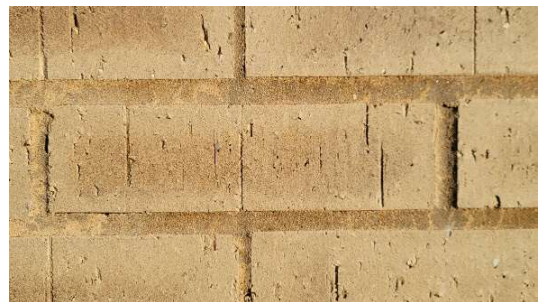
Photo #91: Close-up view of brick discoloration (south elevation, stairwell, 1/12/22).
