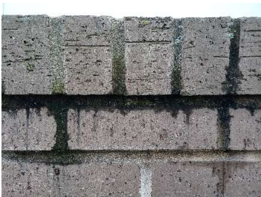
Photo #93: Close-up view of dark residue on the mortar (north elevation, gymnasium, 1/12/22).
