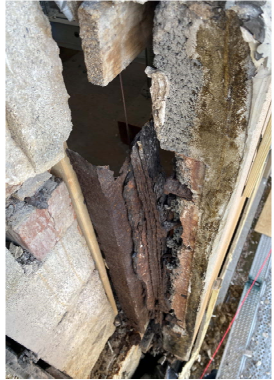
10. Severe corrosion of steel connections. Image taken from exterior after column was demolished.
