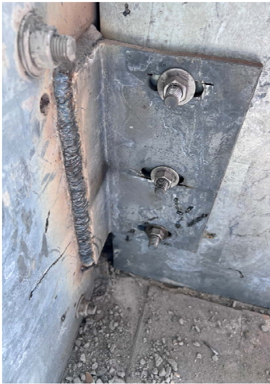
15. New connection includes slotted holes, enabling thermal movement of the precast panels.
