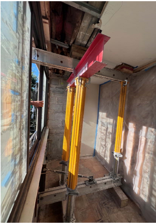
11. Shoring with turnbuckle device. Note the construction barrier/demising wall separating the bedroom from the work zone.
