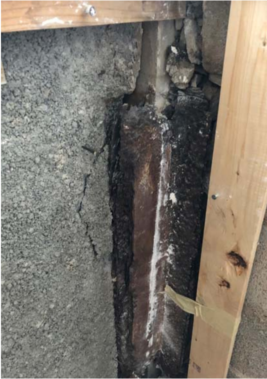
9. Severe corrosion of steel connections. Image from interior showing disengagement.
