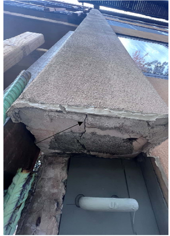
12. Cracks hidden by the coating.
