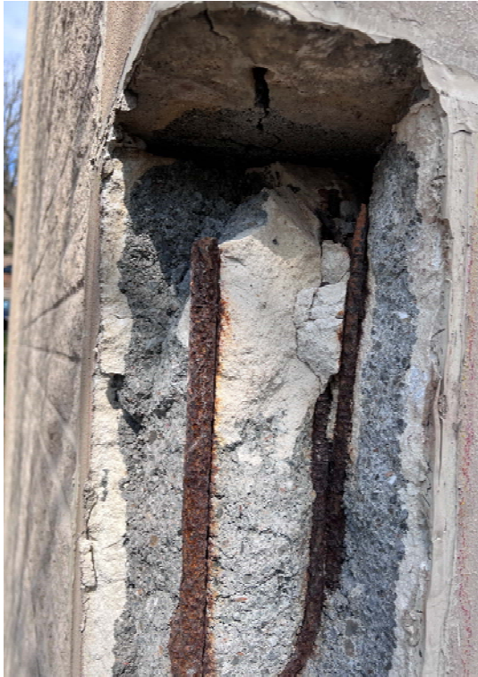
13. The concrete column profile and sever corrosion of rebars.
