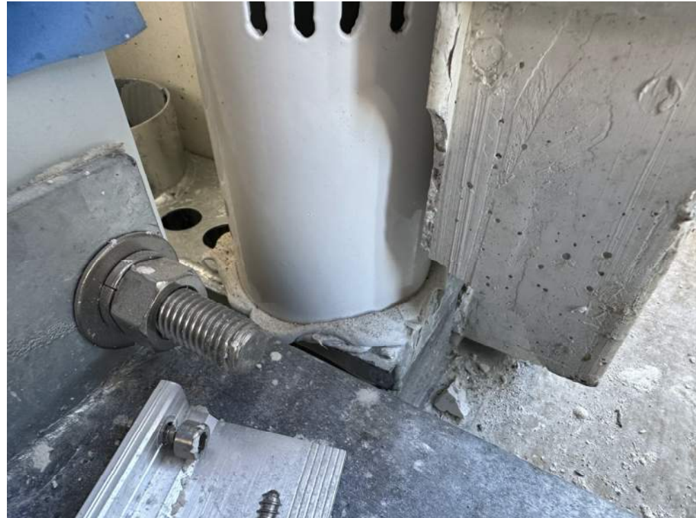
Steel duct set in sealant and sealed to HDG duct extension
