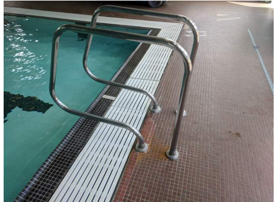
Original 30+ year old handrails, good condition
