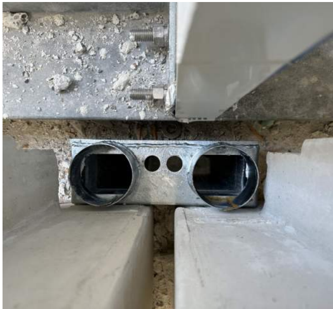
HDG duct adapter set in sealant
