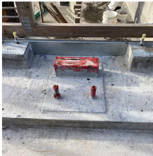
Bolts fully welded and duct extension raises connection above the plane of drainage
