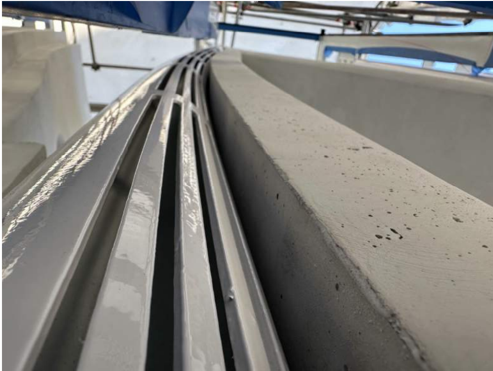
Diffusers located based on CFD
