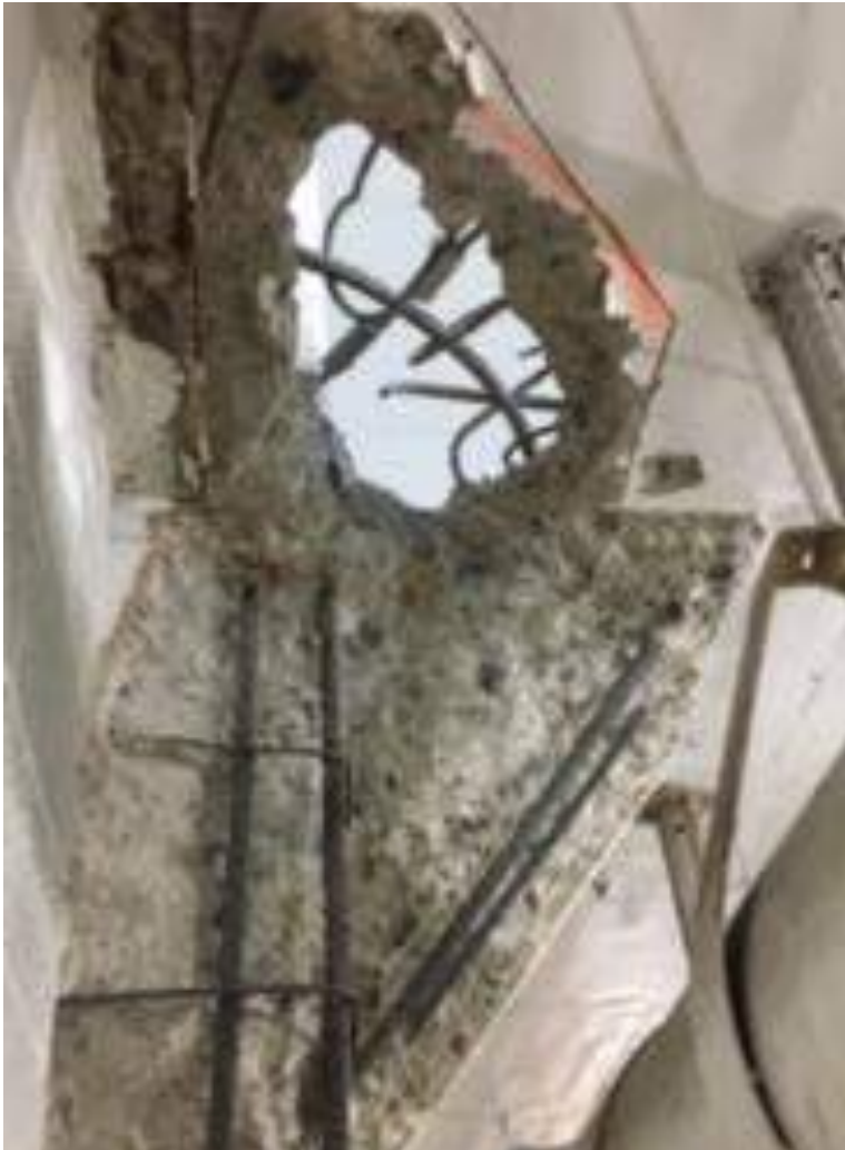
CORBEL AND COLUMN REPAIRS
