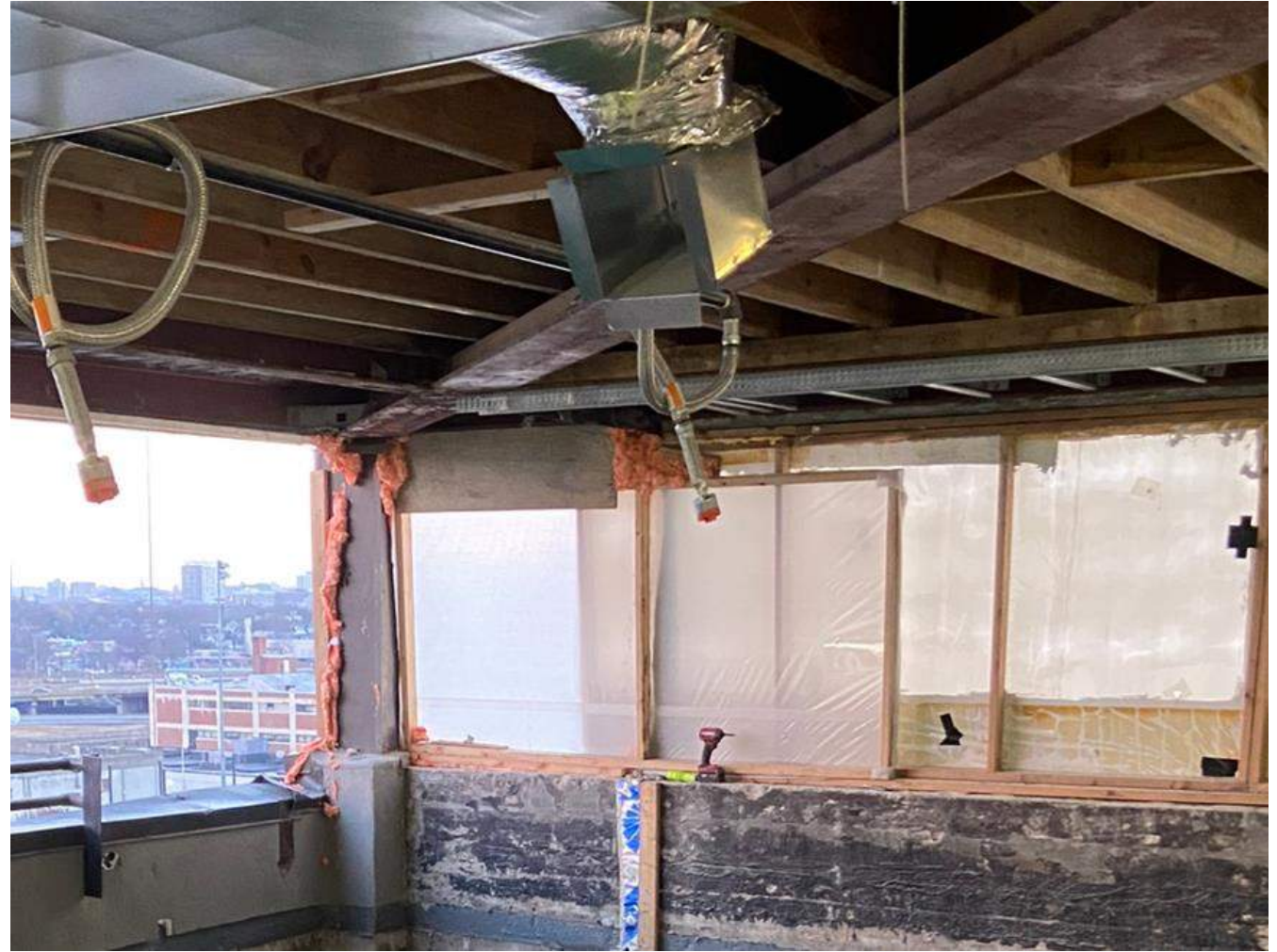
WOOD-AND-STEEL-FRAMED ADDITION
