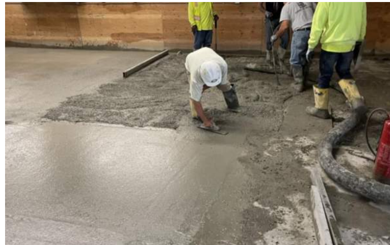
LARGE TOPSIDE NEG. MOMENT REPAIRS
