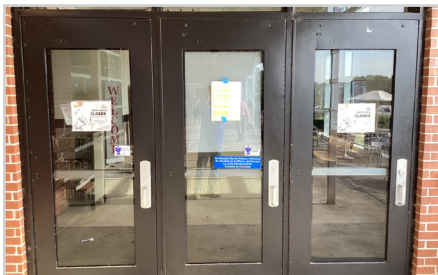
2015 Exterior Doors (Hollow Metal)
