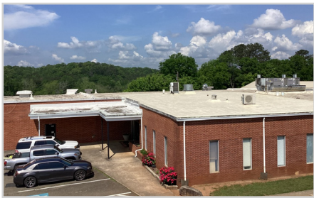
2061 Roof (Modified Bitumen)
