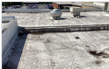
2014 Roof (Modified Bitumen)
