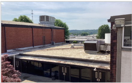
2040 Roof (Polyurethane Foam)
