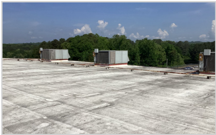
2080 Roof (Modified Bitumen)
