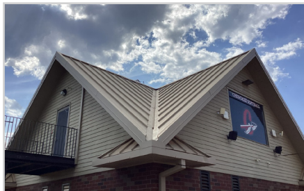
Softball Pressbox Roof (Standing Seam Metal)
