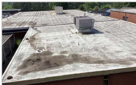
2020 Roof (Modified Bitumen)
