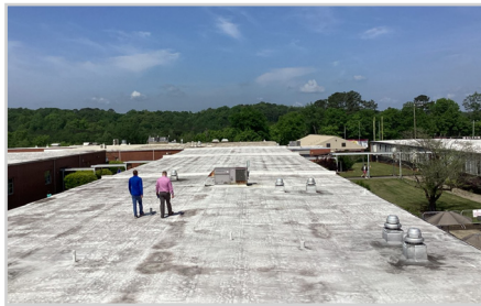
2012 Roof (Modified Bitumen)
