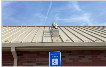
Field House Roof (Standing Seam Metal)
