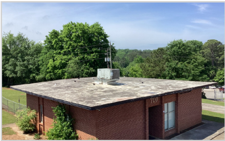
2070 Roof (Modified Bitumen)
