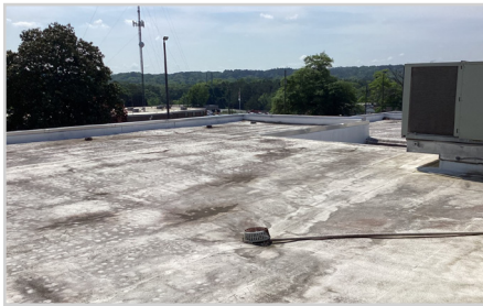
2012 Roof (Modified Bitumen)
