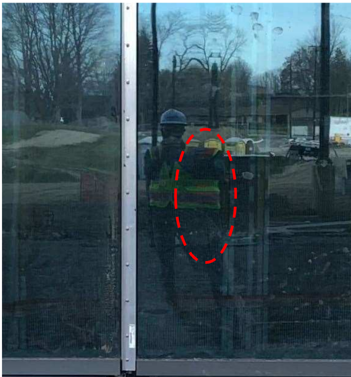
Photo #2: Distorted reflected image of a person after moving slightly towards the right.
