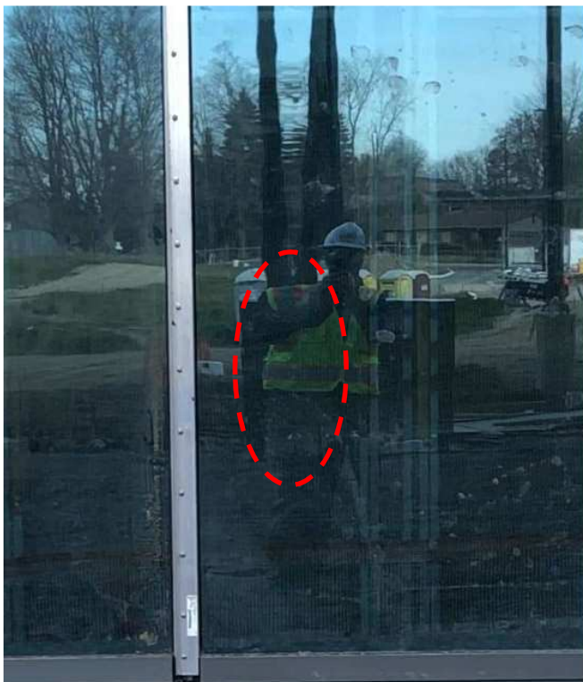
Photo #4: Distorted reflected image of a person after moving slightly further towards the right.
