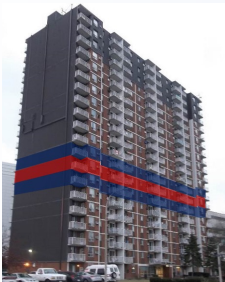
PHOTOGRAPH 7. Sample of guarding for a whole-floor test, with the test floor in red and the guards in blue.
