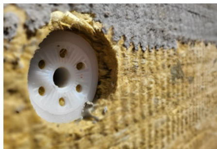
PHOTOGRAPHS 2 & 3. Photographs 2 and 3. Stage 1 fastener through mineral wool insulation, countersunk to allow for insulation plug and stage 2 fasteners installed over the fully cured base coat.
