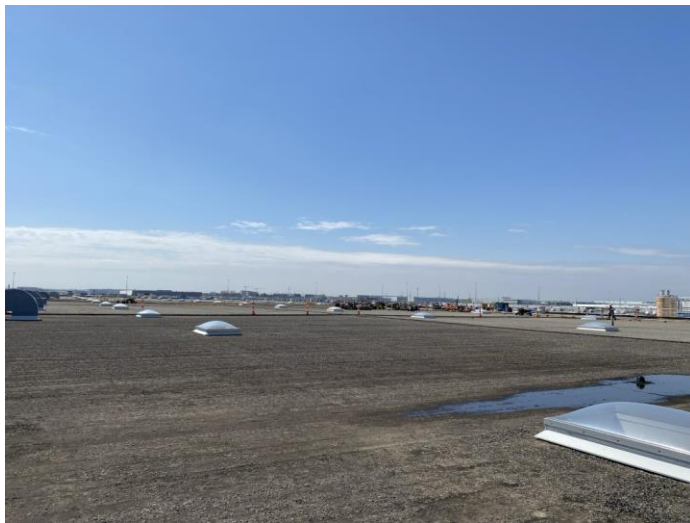
Existing Industrial Building BUR Roof System
