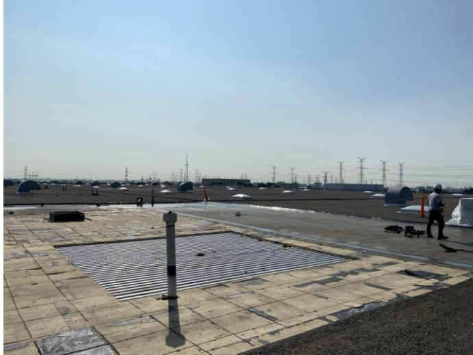
Existing BUR membrane removed and localized ‘wet’ insulation being replaced
